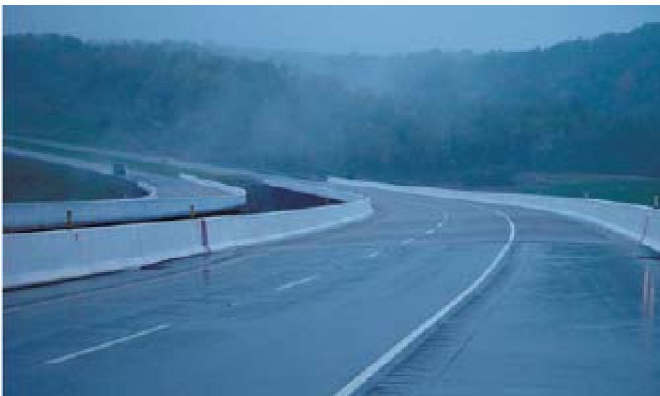
FIGURE 44 White concrete bridge rail.
