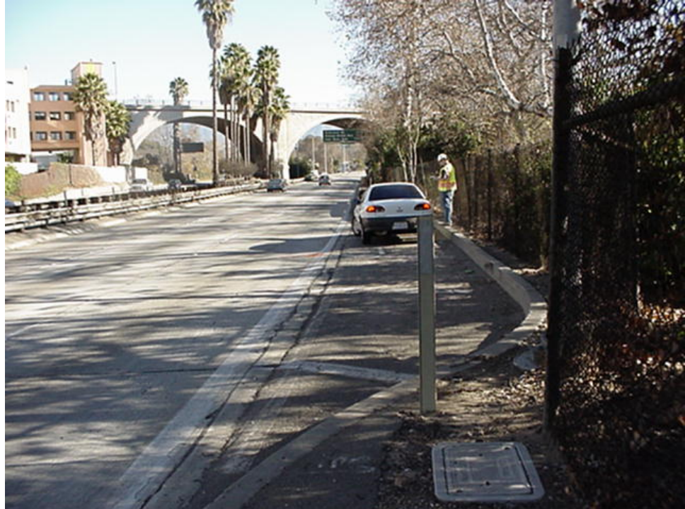
FIGURE 119 Pull-off areas are provided periodically along the outside lanes.
