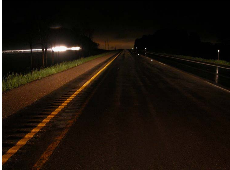
FIGURE 34 Painted edgeline rumble strips.
