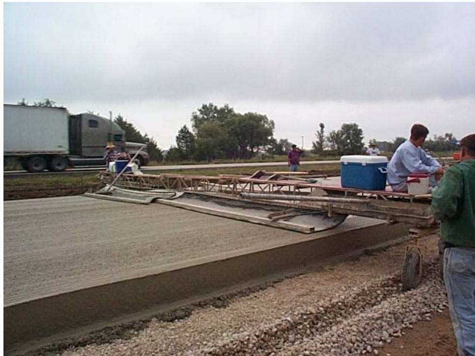
FIGURE 62 Longitudinal texture applied to fresh pavement to improve surface friction.
