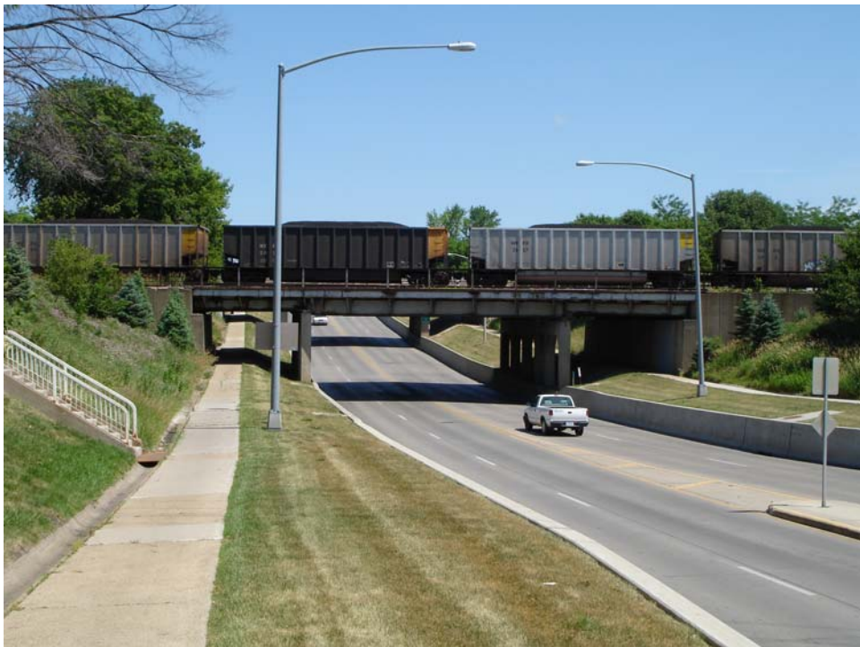
FIGURE 19 Sight distance at an undercrossing.
