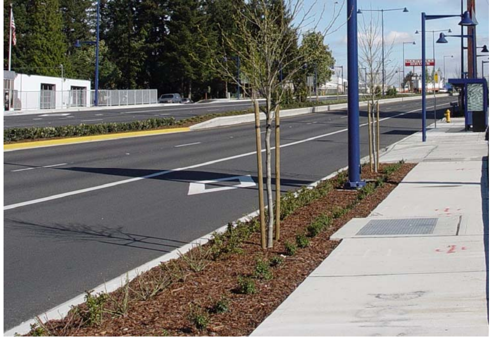
FIGURE 109 Sloped-down end section adjacent to turn lane.
