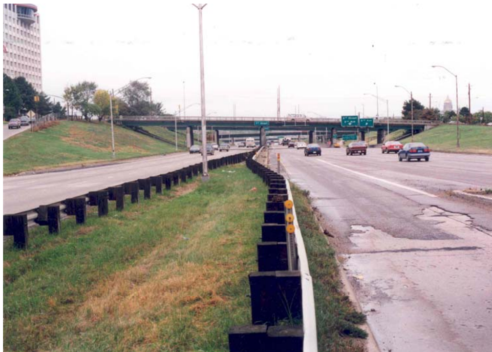
FIGURE 72 Interstate 235 before reconstruction.
