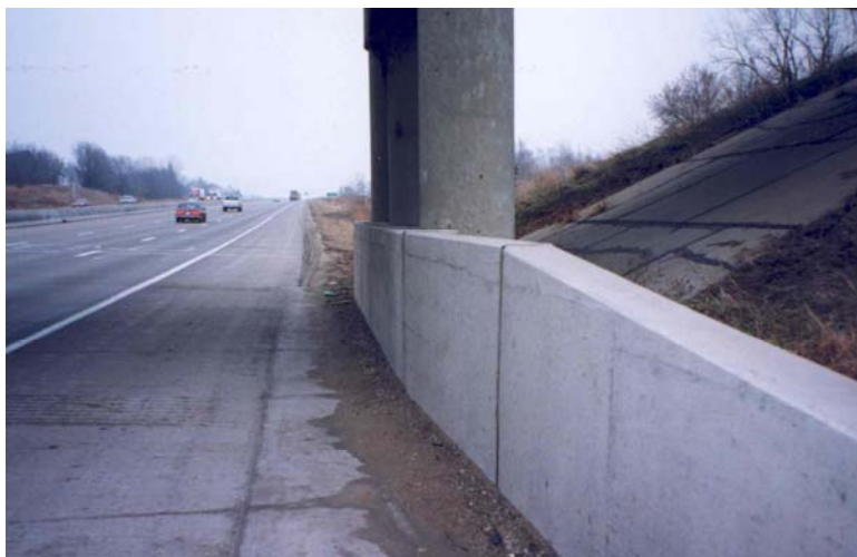
FIGURE 39 Shielding fixed objects with barrier.
