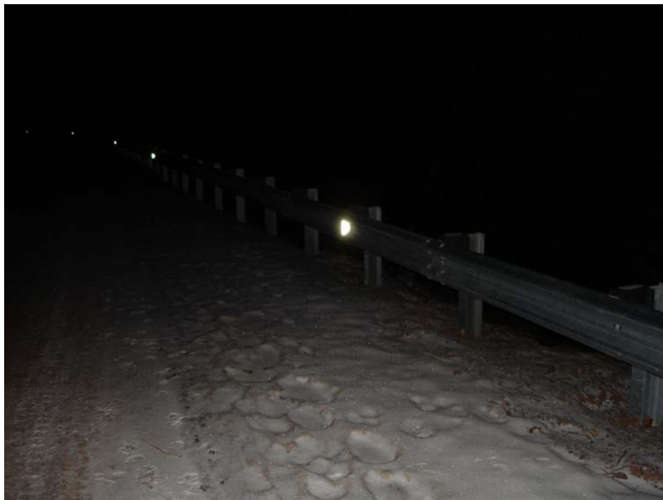
FIGURE 52 Delineation with reflectors on barrier.
