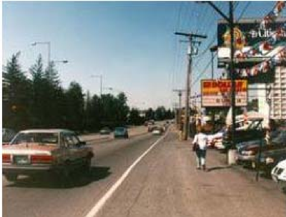
FIGURE 99 SR 99 before reconstruction in SeaTac (top) and Shoreline (bottom). Note the wide paved shoulders, lack of access control, and no sidewalks. One of the primary goals of the communities along the highway was to create a more attractive, pedestrian- friendly local environment.
