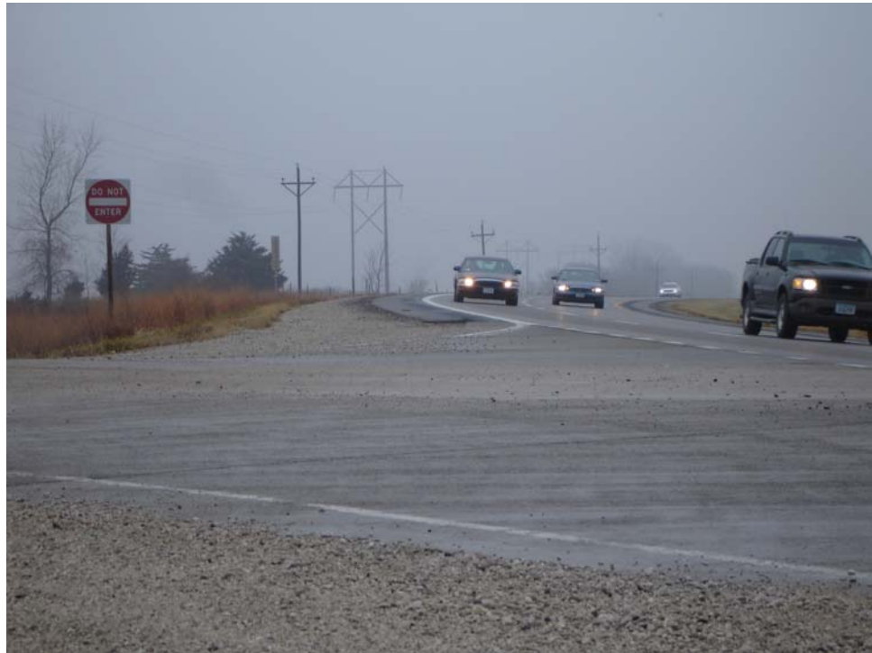
FIGURE 15 Superelevation
