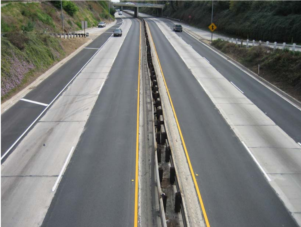
FIGURE 120 Enhanced delineation with raised pavement markers and pavement markings with high retroreflectivity. Reflectors will also be placed along the new concrete median barrier.
