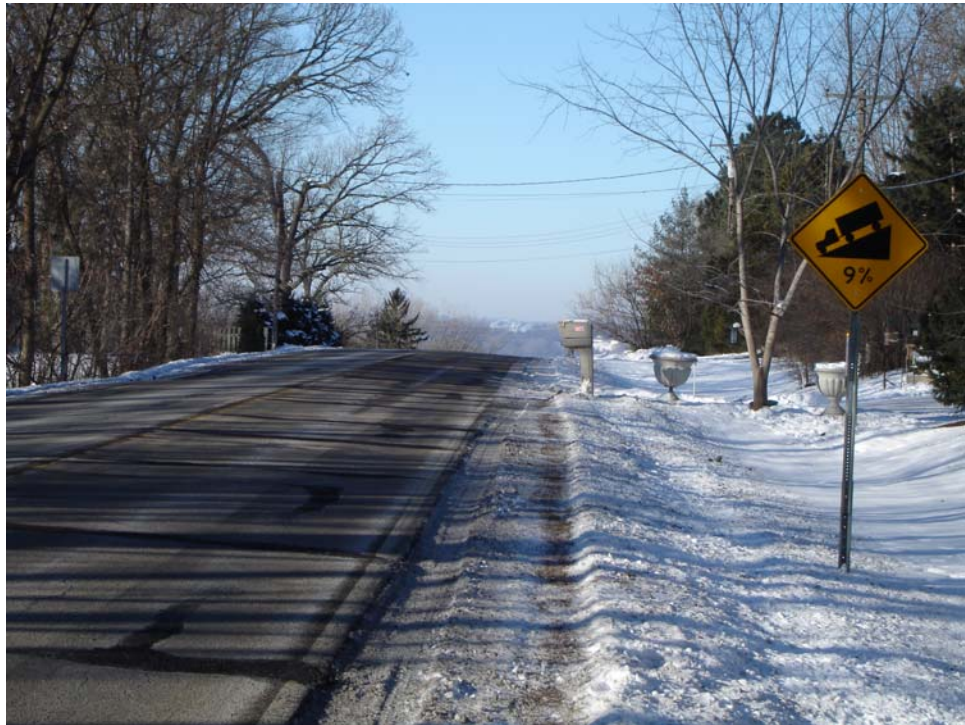
FIGURE 53 Advance warning of a steep grade.
