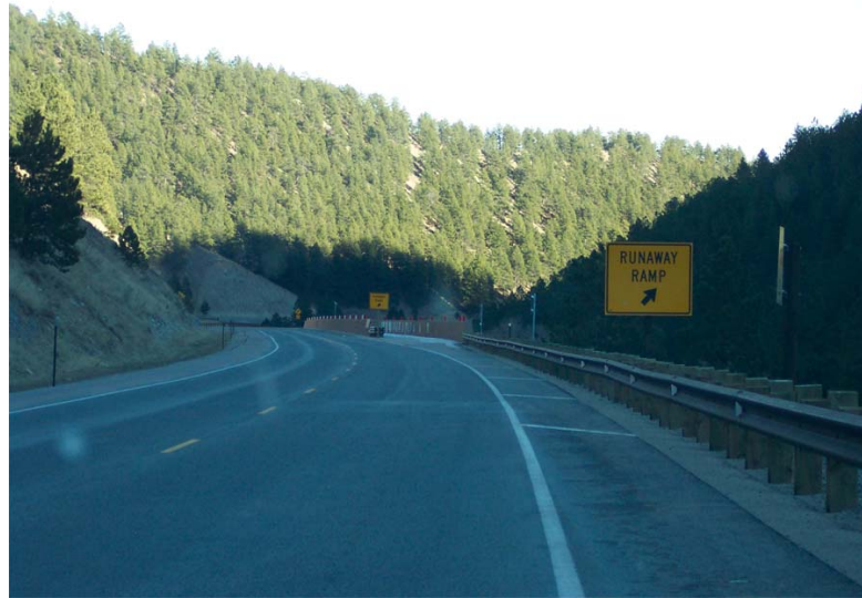
FIGURE 92 Runaway truck ramp. A nearby ramp on the other side of the roadway was replaced because it required crossing the opposing lane of traffic.
