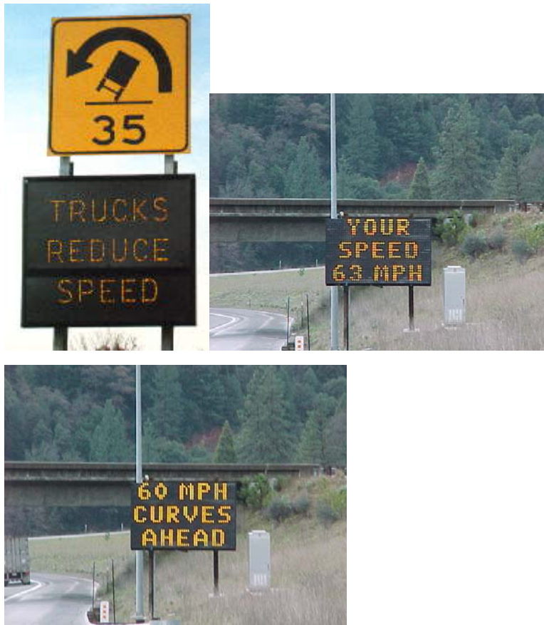
FIGURE 49 Dynamic curve warning system.
