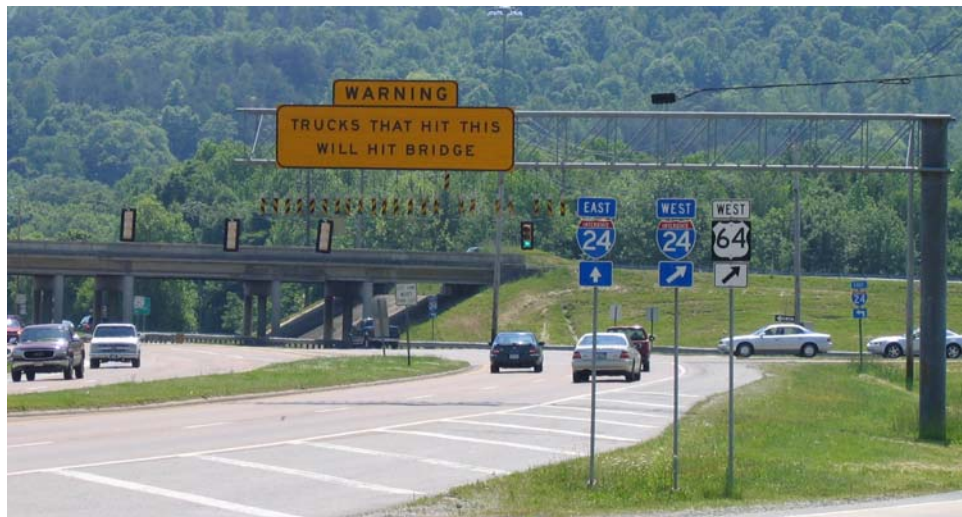
FIGURE 67 Warning sign with hanging chimes installed at the same height as the vertical clearance of the structure.
