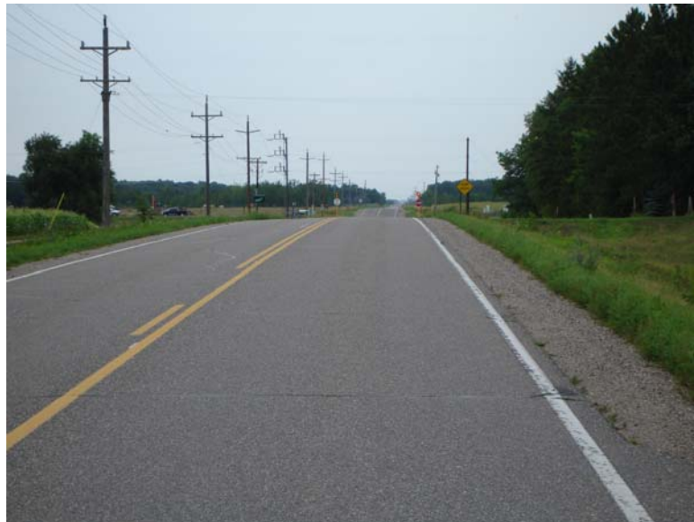
FIGURE 59 A STOP sign with a flashing beacon improves visibility of the sign at this intersection with limited vertical sight distance.
