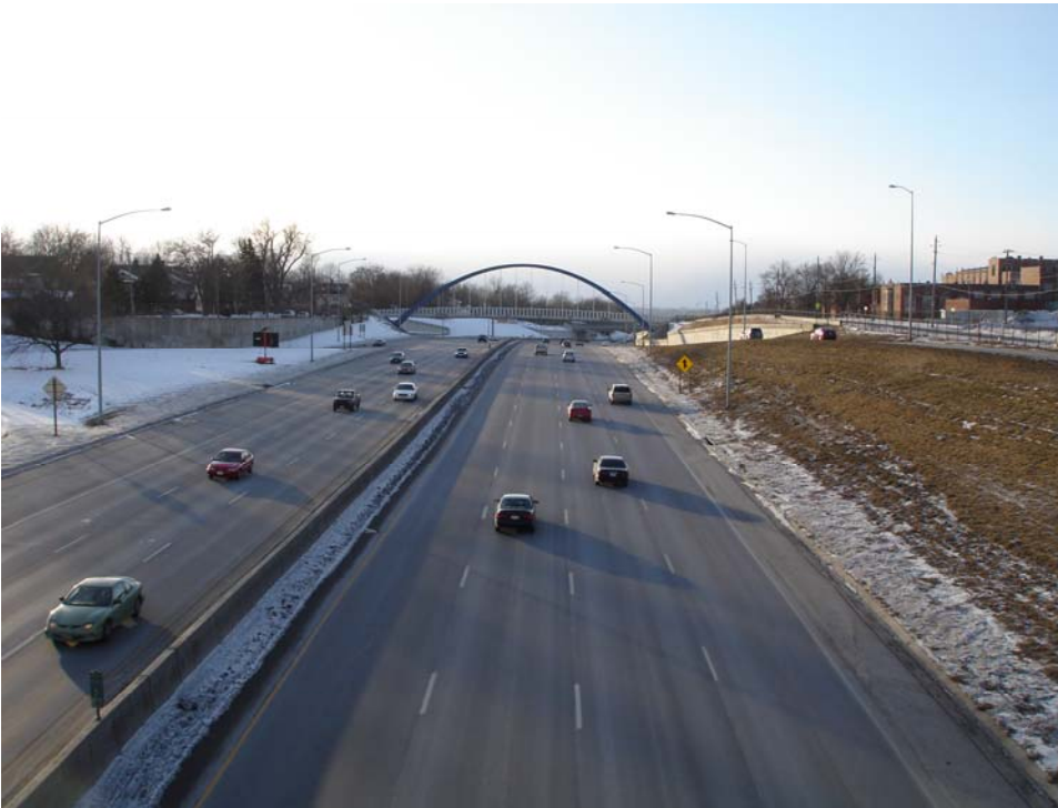
FIGURE 73 Interstate 235 after reconstruction.
