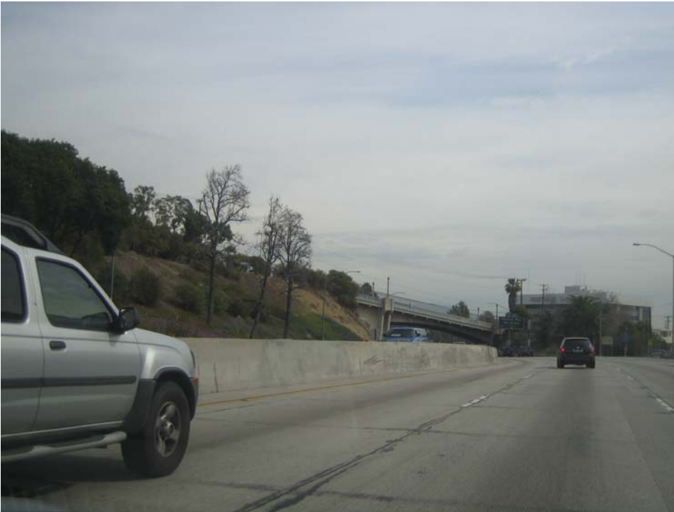
FIGURE 118 Single-slope concrete median barrier at a horizontal curve.
