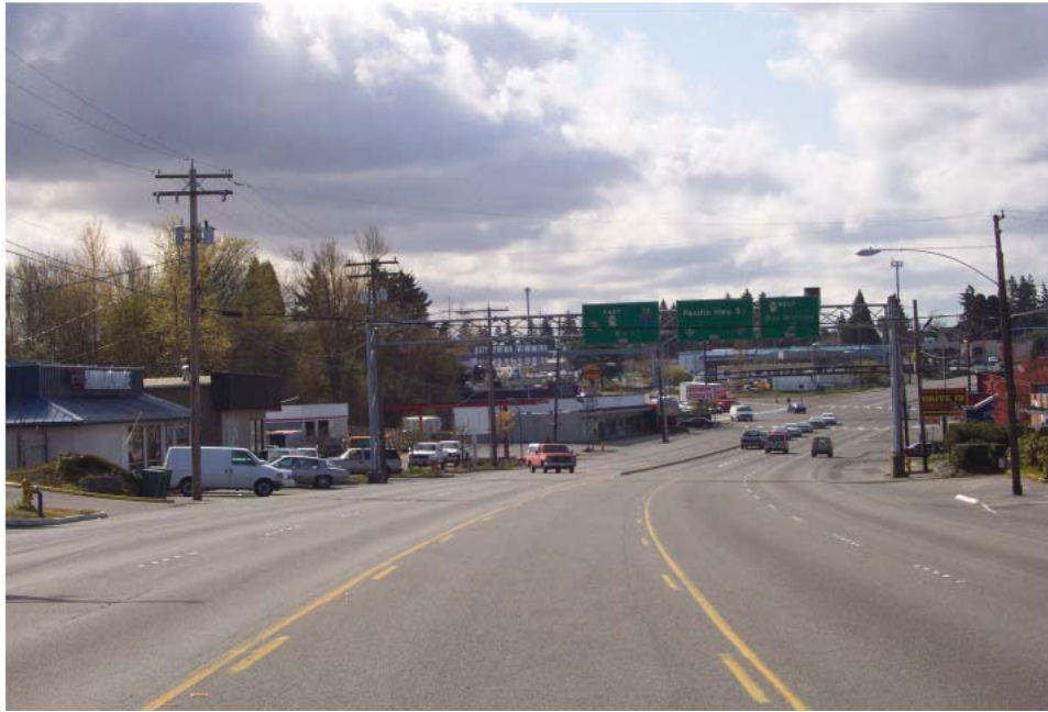
FIGURE 98 SR 99 before and after reconstruction in Des Moines. The five-lane cross section with a two- way left-turn lane was common throughout the corridor.
