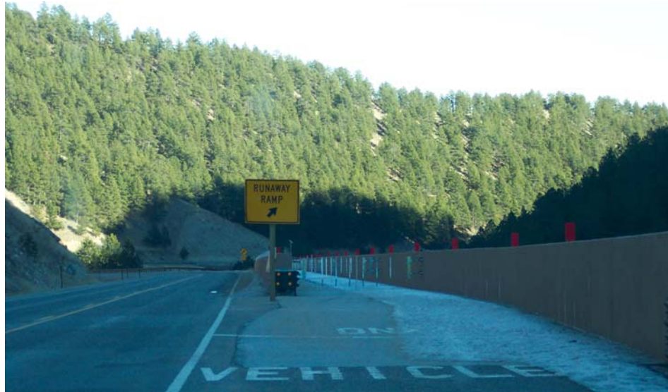
FIGURE 55 Truck escape ramp.
