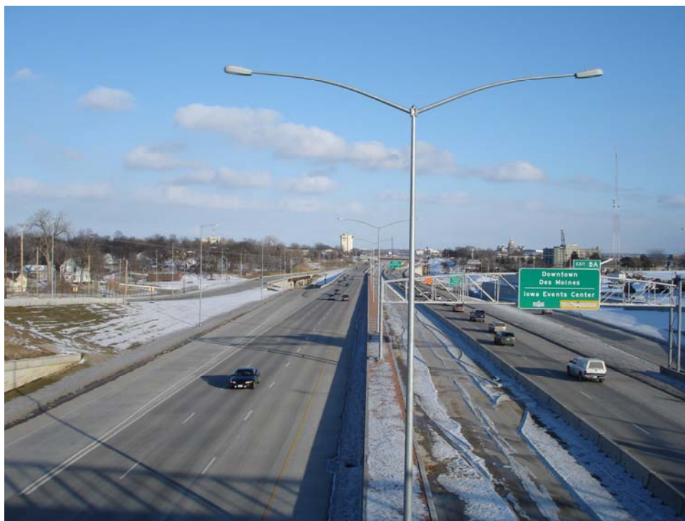
FIGURE 80 Lighting was placed down the center of the median where more cross-sectional width was available.
