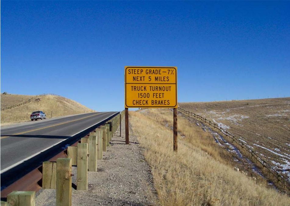
FIGURE 89 Advance signing for the brake-check turnout.
