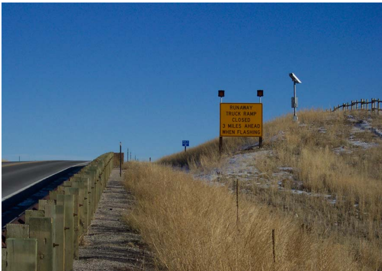
FIGURE 93 Electronic signing provides advance warning when the truck ramp is closed.
