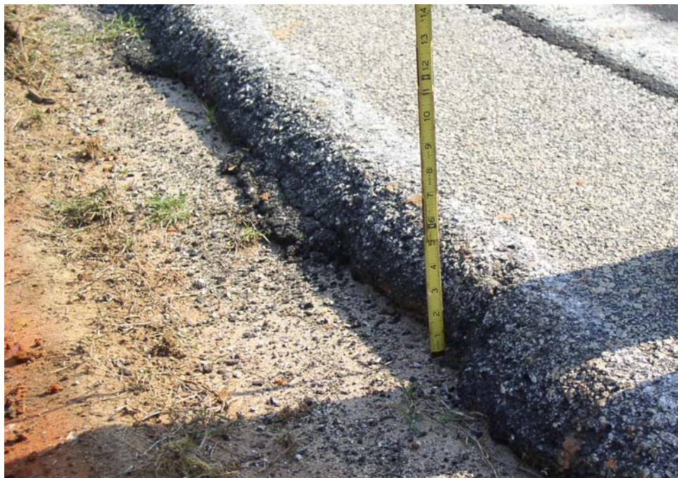
FIGURE 9 Pavement edge drop-off.
