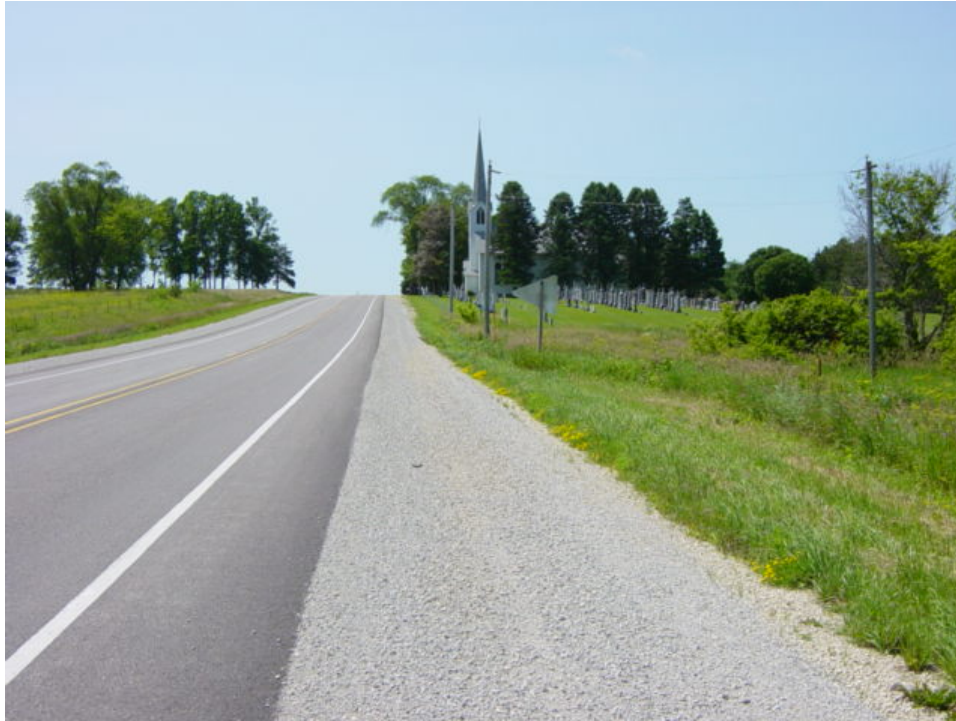
FIGURE 9 Pavement edge drop-off.
