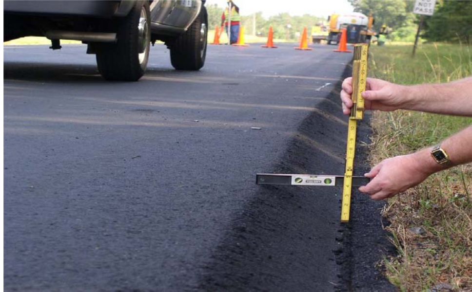
FIGURE 36 Safety edge (top) and after the shoulder has been graded over the edge (bottom).
