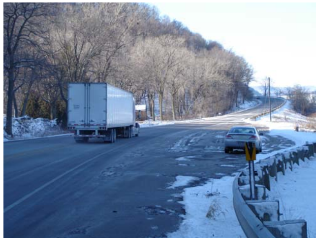
FIGURE 40 Pull-off area on the inside of a horizontal curve.
