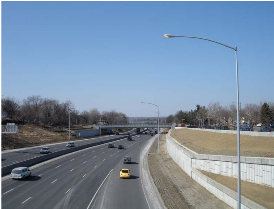
FIGURE 79 Lighting was placed on the outside of the freeway through the design exception area.
