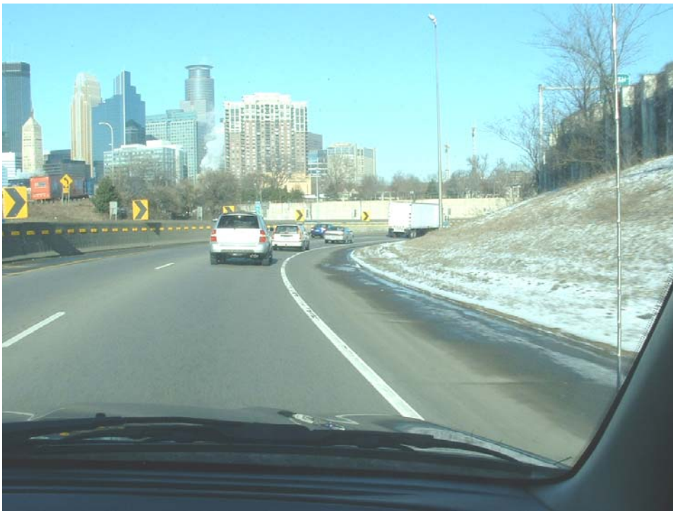
FIGURE 50 Delineation with large chevrons.
