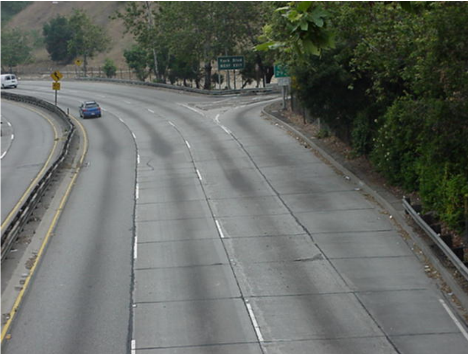
FIGURE 116 The Arroyo Seco Parkway has a narrow cross section, a curvilinear alignment, and non-standard interchange geometry.
