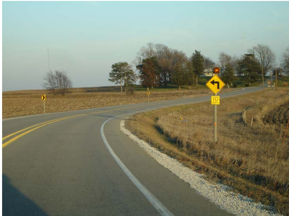
FIGURE 47 Turn warning sign with flashing beacon.
