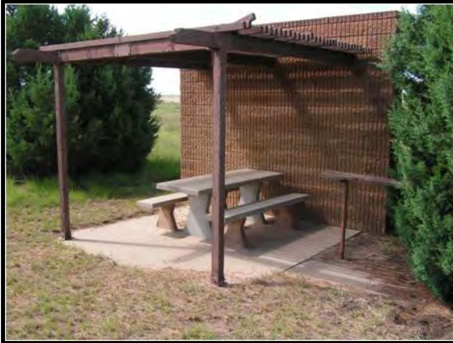
Failing dangerous overhead canopy and wall of table shelter removed with the table left in place for public use
