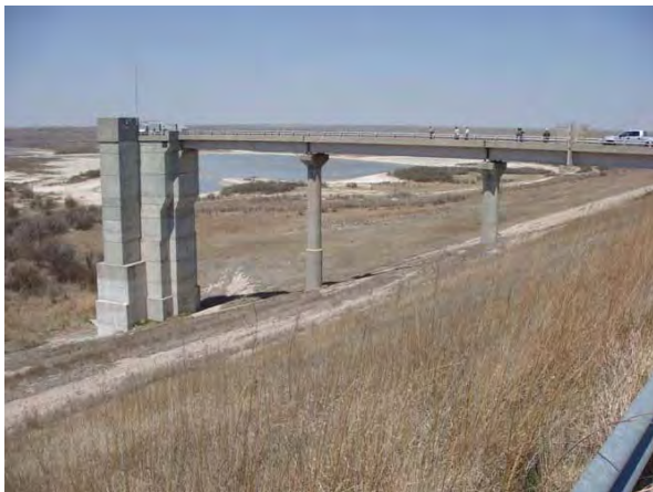
Outlet Works and Gate Tower
