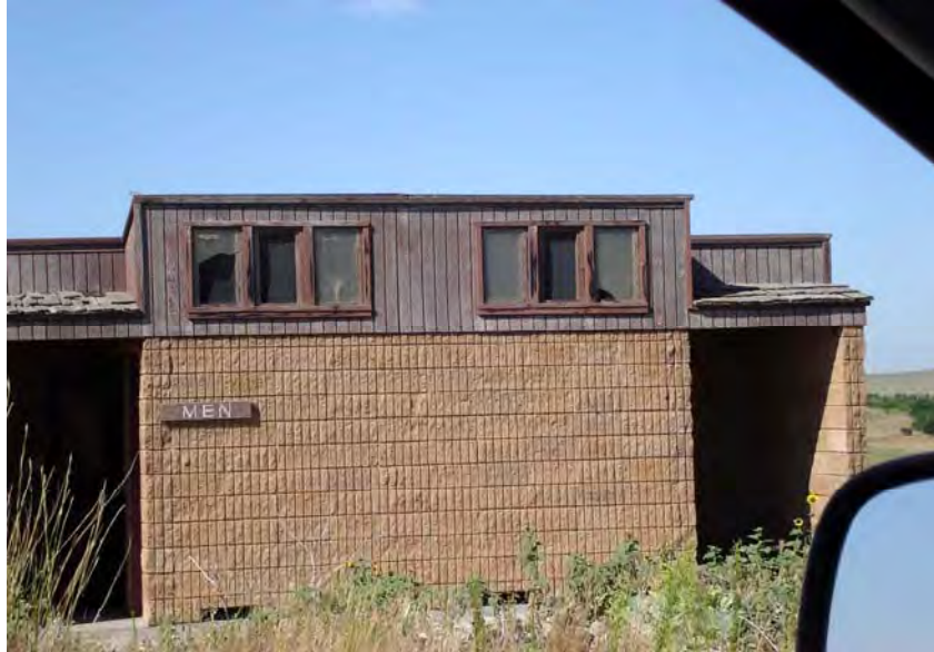
Figure 2-5 Example of a Typical Restroom Structure
