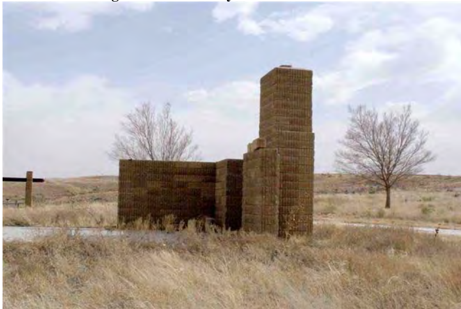
Figure 2-8 Chimney Structure Remnants
