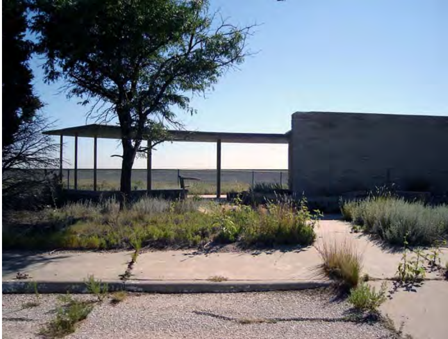
Figure 2-7 Overlook Building and Shelter
