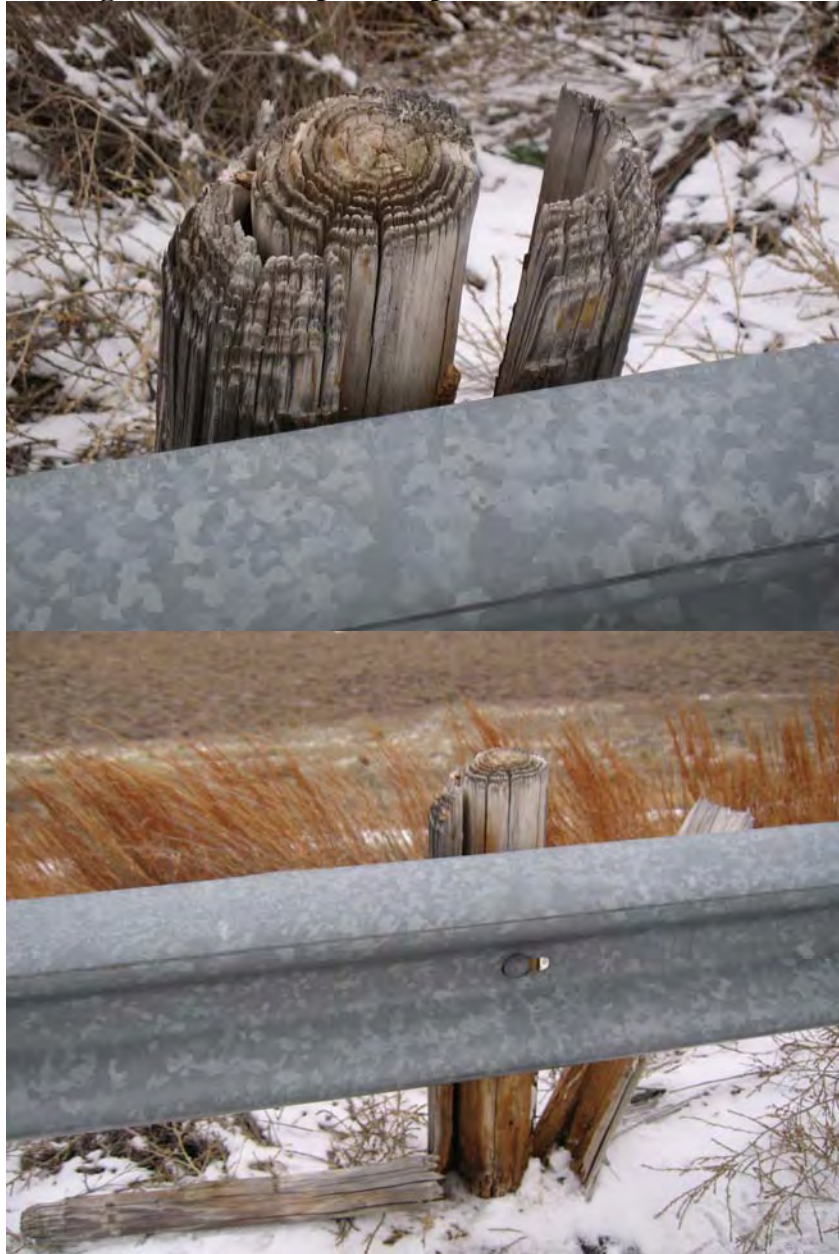
Figure 1-4 Examples of Splintered Guardrail Posts
