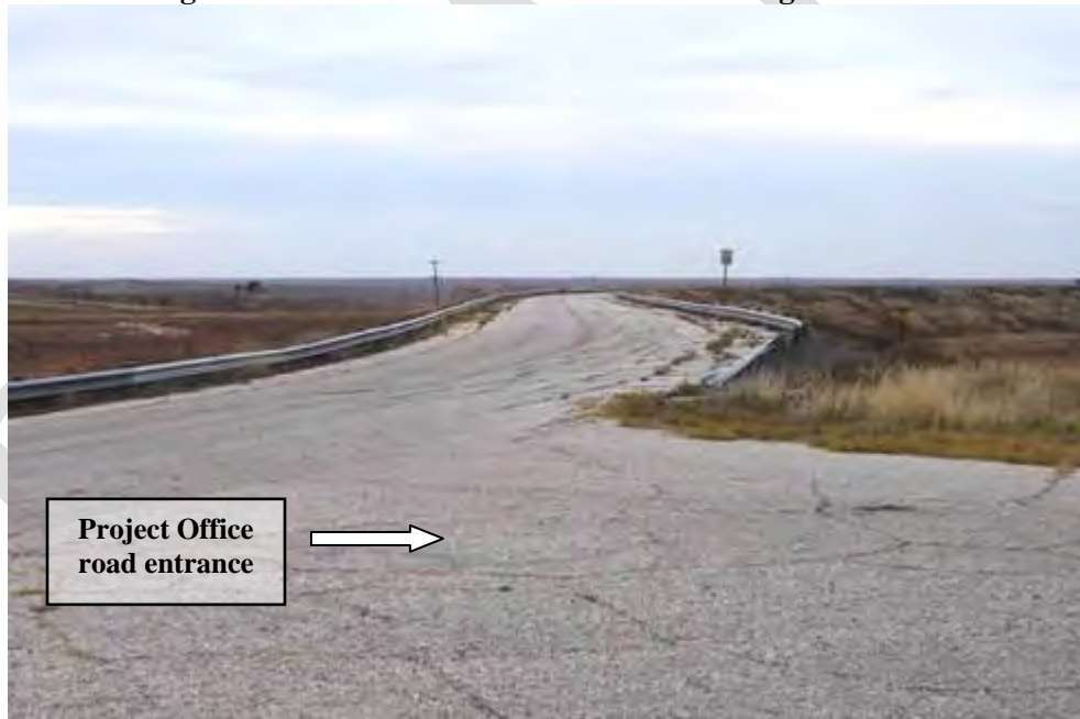
Figure 2-2 View of South End of Road Facing Northwest
