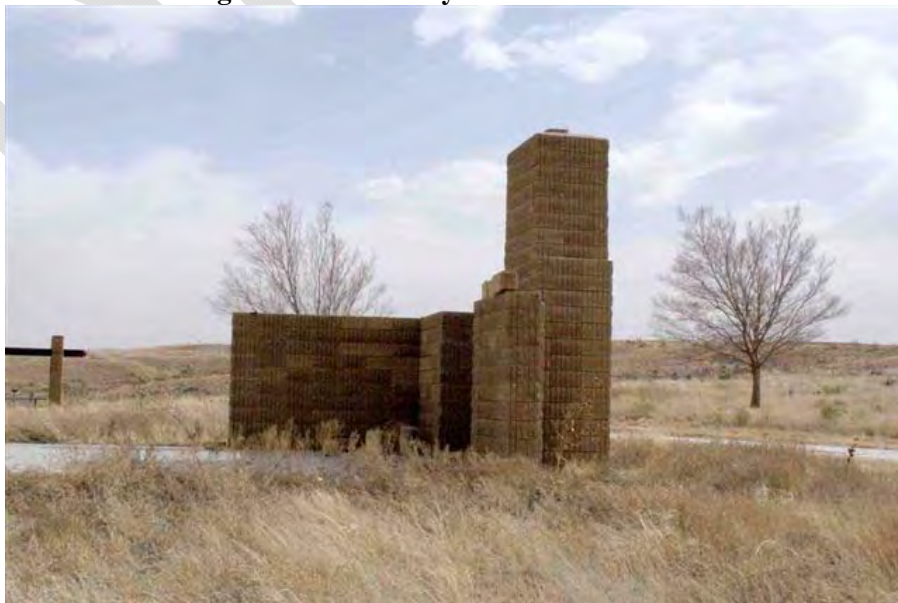
Figure 2-8 Chimney Structure Remnants
