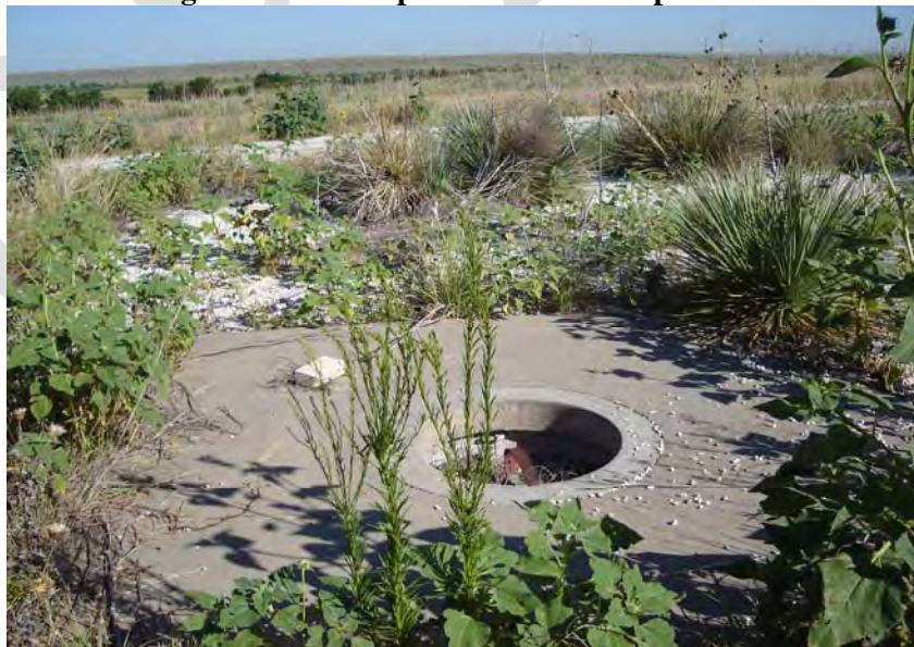
Figure 2-6 Example of Trailer Dump Station
