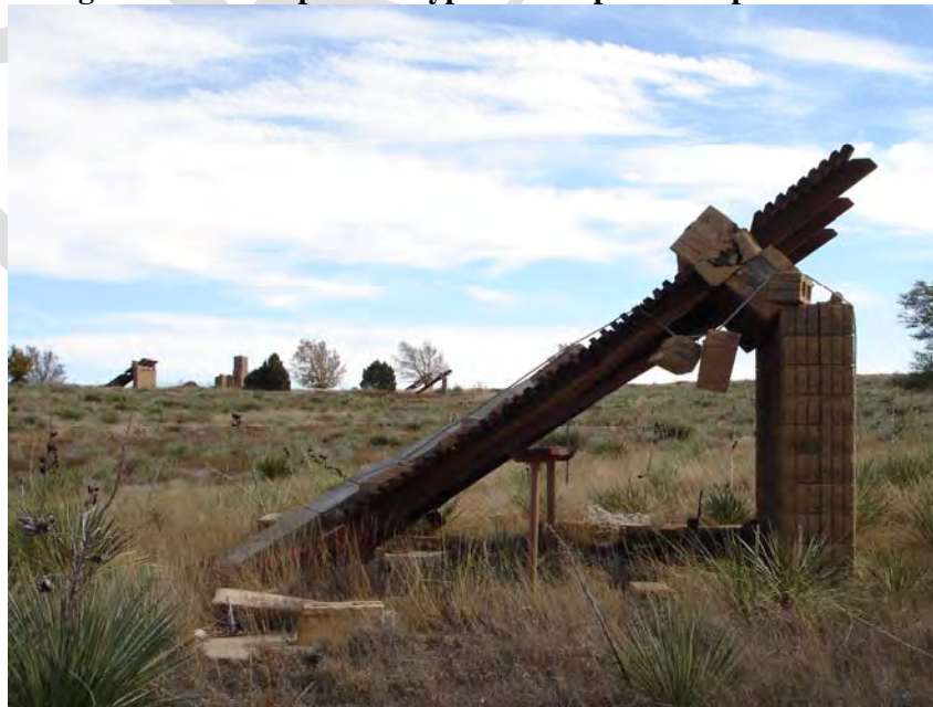
Figure 2-4 Example of a Typical Collapsed Campsite Shelter
