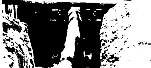
Top left: Impact mole just before connection to HDPE pipe, showing air line inside HDPE pipe. Bottom left: Impact mole bursts a cast iron pipe and forces it into the surrounding soil. Above: HDPE pipe is inserted into the pit.
