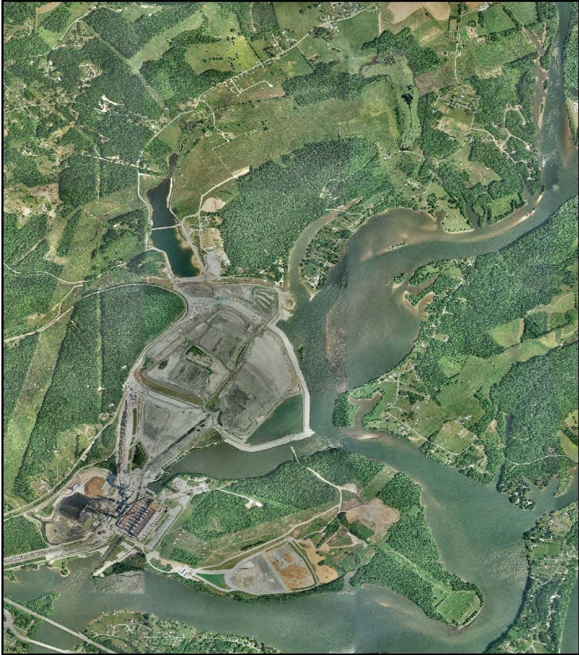
Aerial Image of Kingston Ash Slide (05/02/2012)
