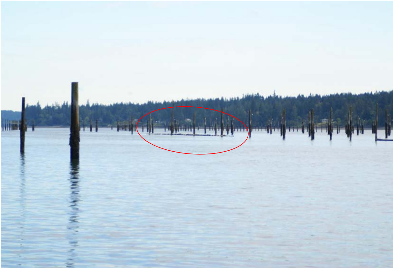
Figure 2: Example of Piling Field and Haul-out Area in Henderson Inlet.
