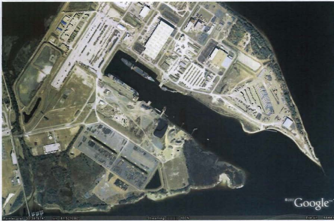
Figure 3 - Close up of MSCF-BI slipway
