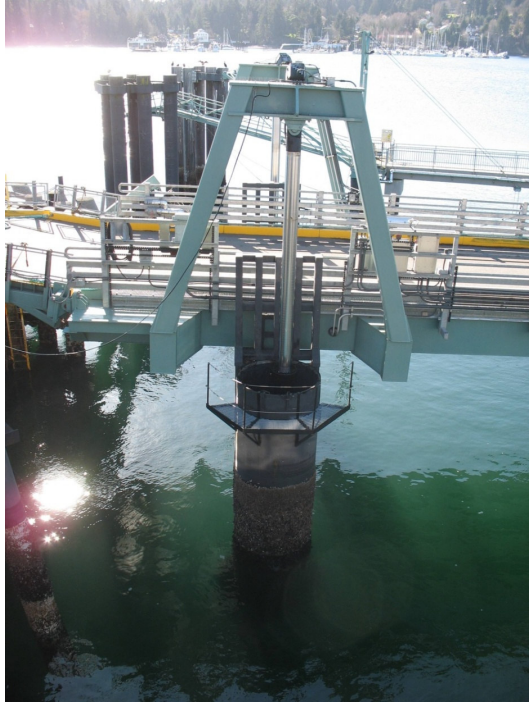
Figure 1-4. Bainbridge Ferry Terminal Transfer Span and Hydraulic Tower
