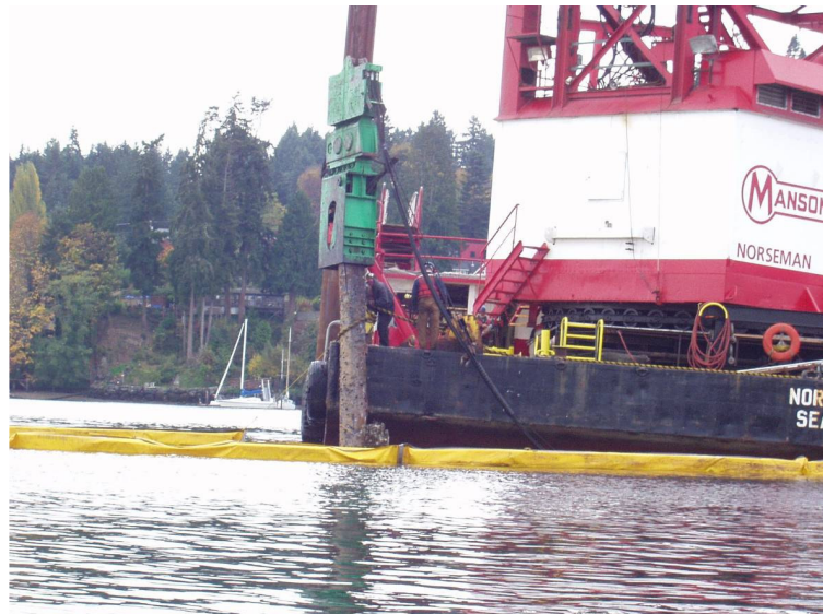
Figure 1-7. Vibratory Hammer Removing a Timber Pile
