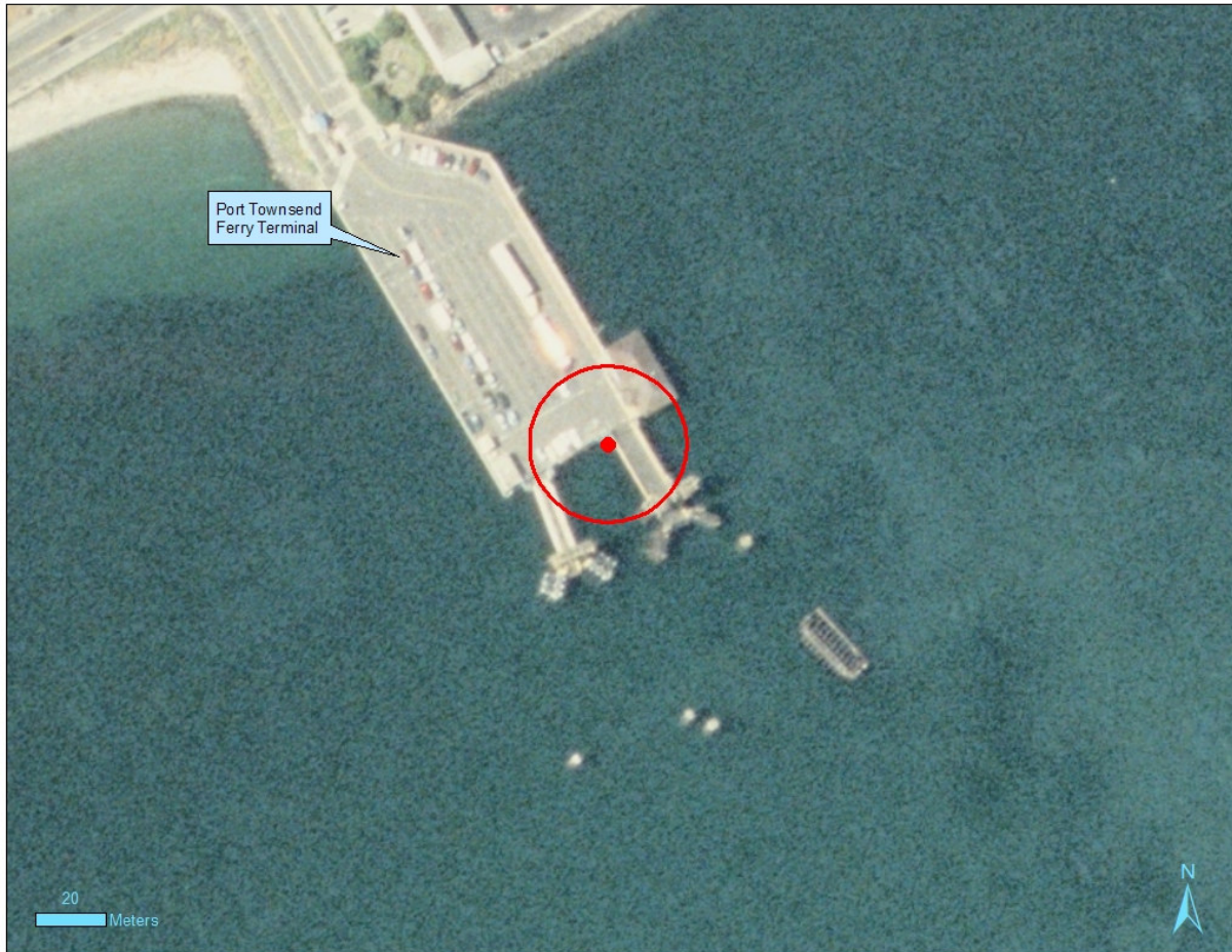
Figure 1 – Approximate 22 m impact pile driving marine mammal shut-down safety zone.
