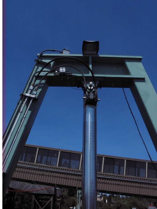
Figure 1-5. Bainbridge Ferry Terminal Hydraulic Tower
