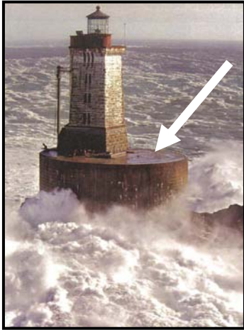
Figure 3. Helicopter landing area on St. George Reef Light Station.
