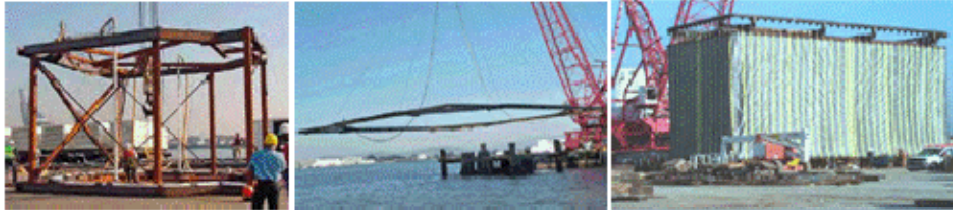
Figure 11-2. Representative large engineering scale air curtain bubble screens not applicable as ELCAS alternative mitigation measure.
