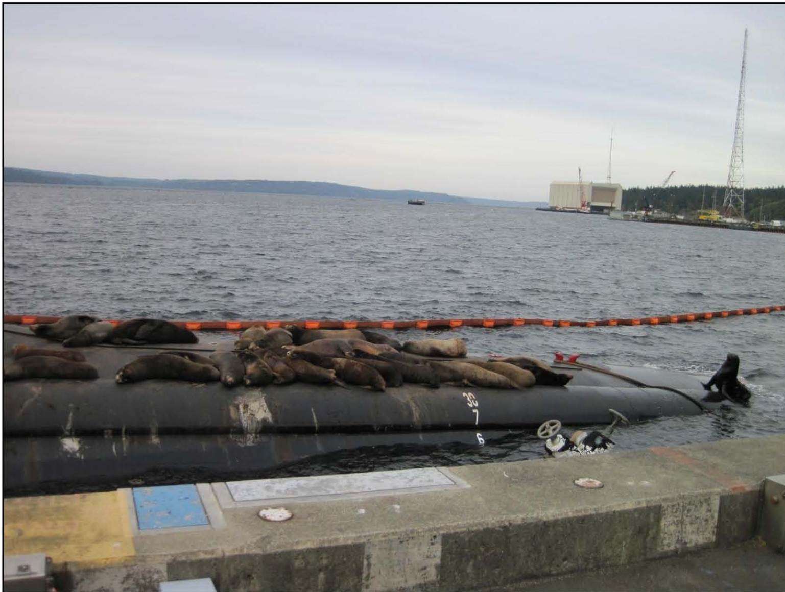
Figure I-2. Delta Pier North, looking towards EHW-1. Photographed 13 October 2011 by A. Balla-Holden, U.S. Navy.
