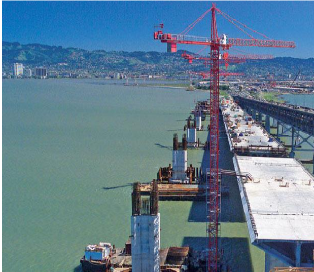
Figure 1-10. Typical Column and Superstructure Construction Using Barge-Mounted Cranes
