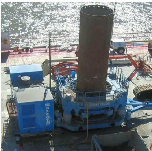
Figure 1-7. Water-Based Drilled Shaft Installation
