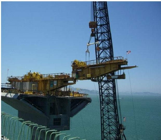
Figure 1-11. Platform-Mounted Crane Placing a Winch on a Superstructure Element
