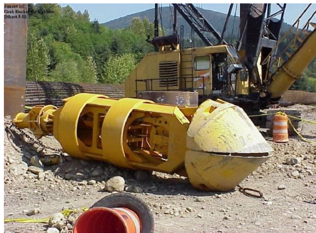
Figure 1-8. Clamshell Used for Removing Material from Drilled Shaft Casing
