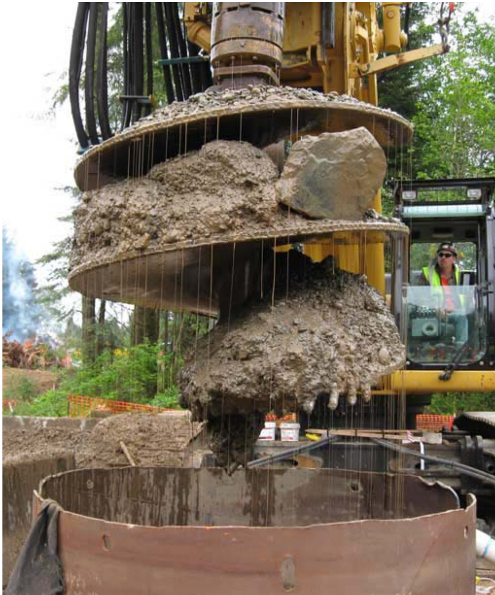
Figure 13 Drilling equipment used to remove soils from a drilled shaft
