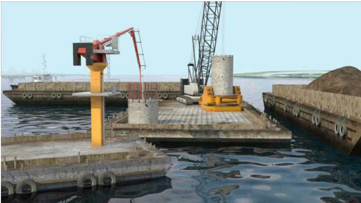
Figure 12 Rendering of an oscillatory equipment setup with concrete, materials, and spoils barges and tug
