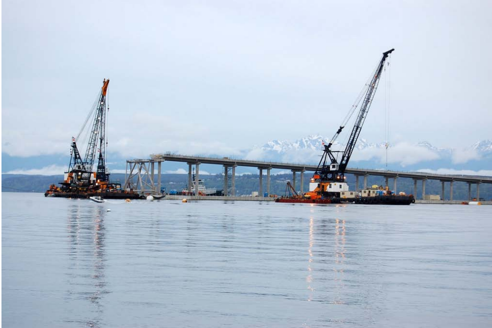
Figure 7 Example of typical barge-mounted construction cranes
