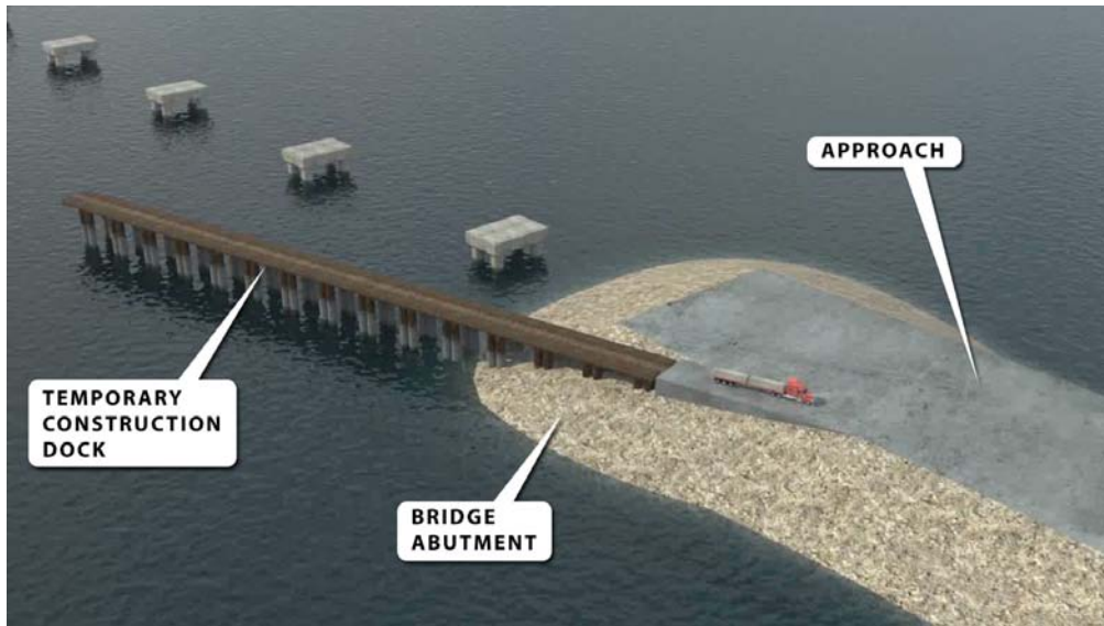
Figure 5 Typical approach showing temporary construction dock at bridge abutments
