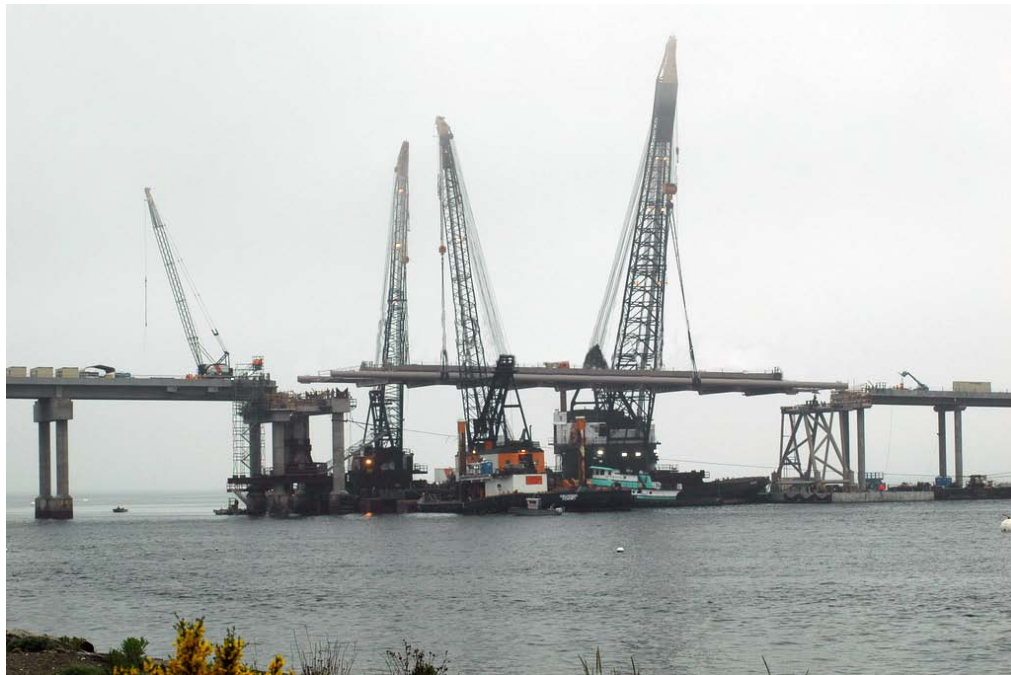
Figure 14 Bridge superstructure lifting and setting by large floating cranes (representative only)
