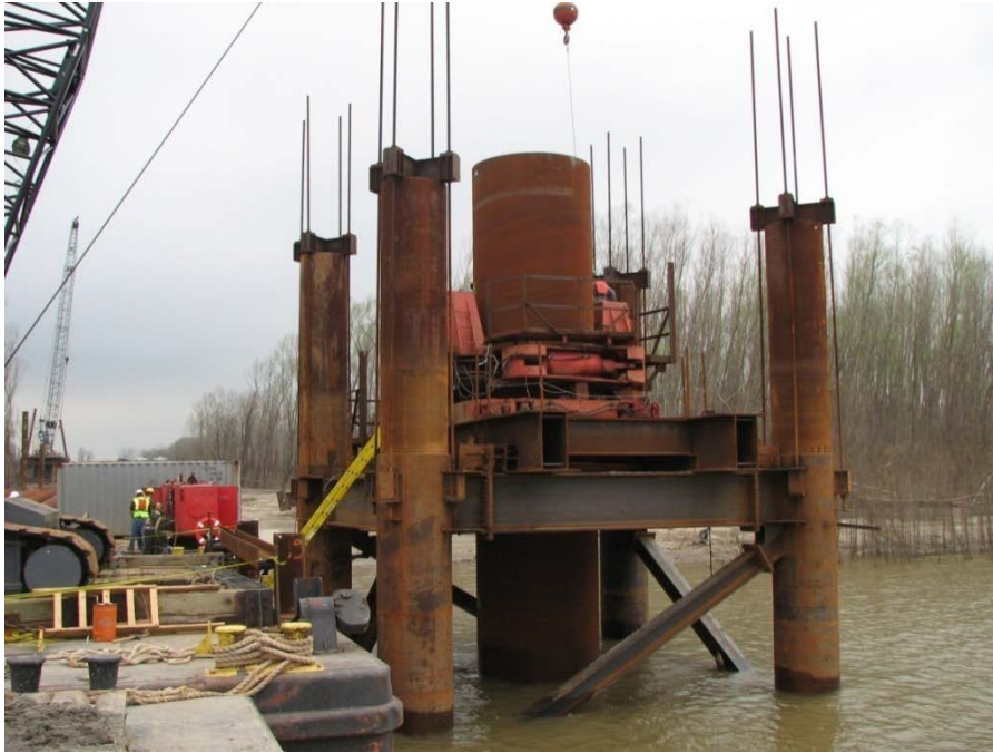
Figure 11 Typical drilled-shaft installation setup
