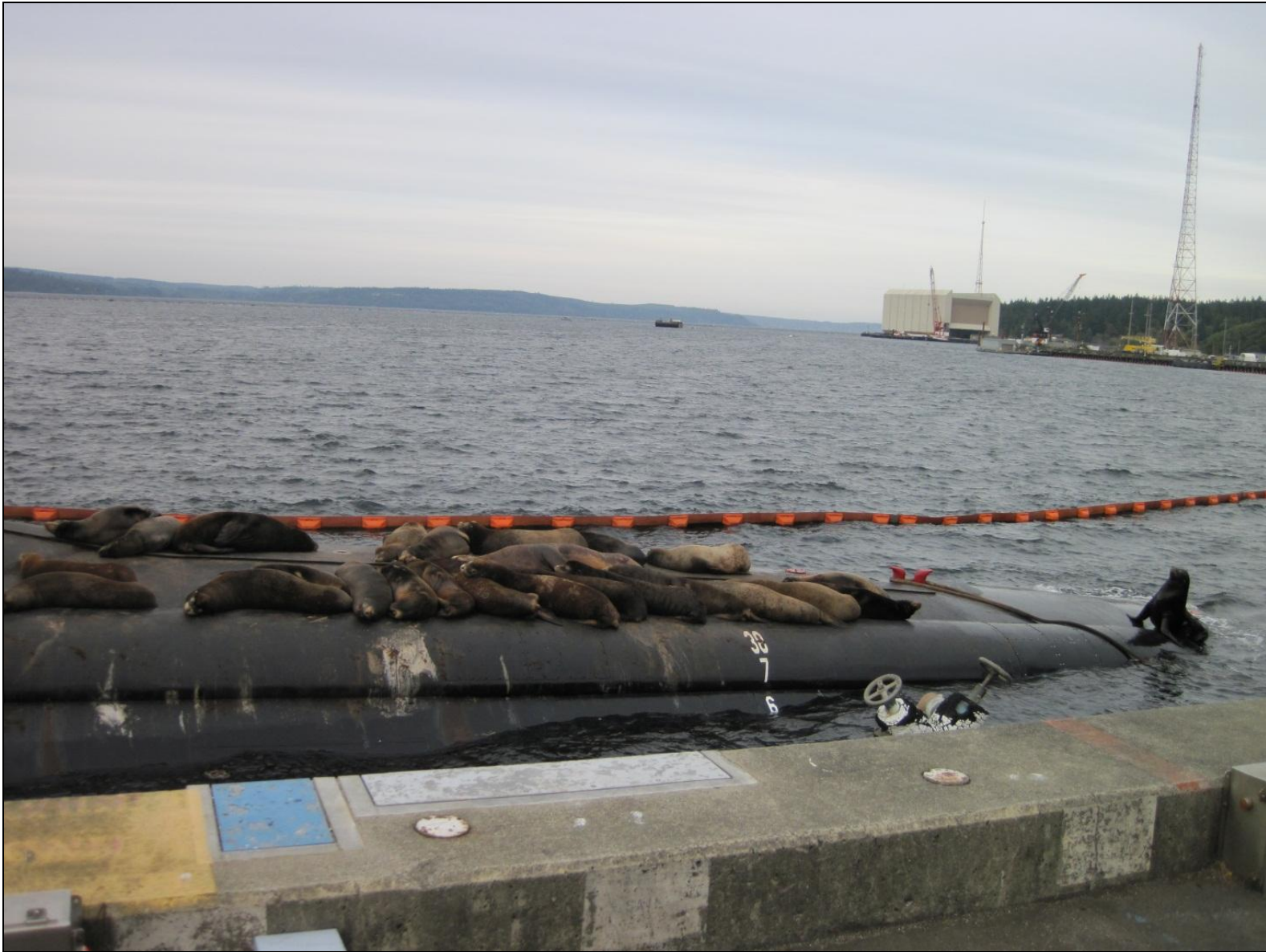
Figure H-2. Delta Pier North, looking towards EHW-1. Photo courtesy of A. Balla-Holden, U.S. Navy.
