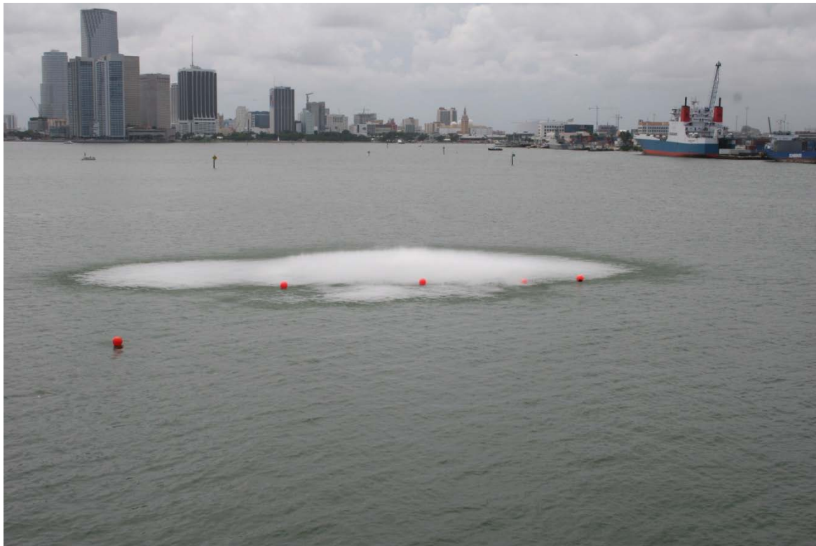
Figure 9 Confined Blast of 3,000 lbs Total Charge Weight of Explosives
