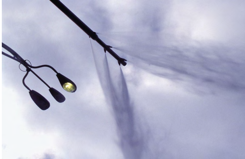
Figure 65. All-Weather Testing Equipment with Experimental Lighting Test Bed Installed on the Smart Road
