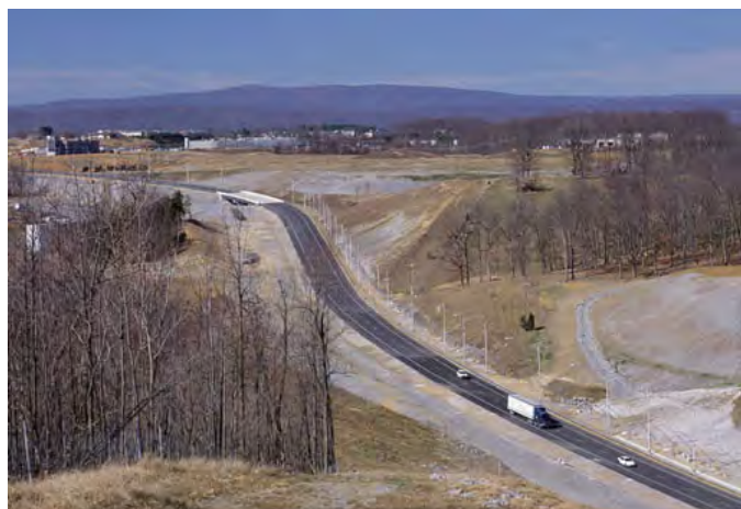
Figure 25. The Virginia Smart Road
