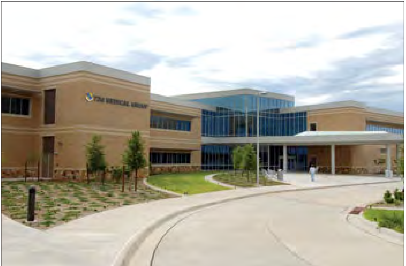
The 72nd Medical Group is another step closer to occupying its new digs. The clinic is located just inside the Gott Gate and will replace the original hospital, Building 5801, that was dedicated in 1960.
