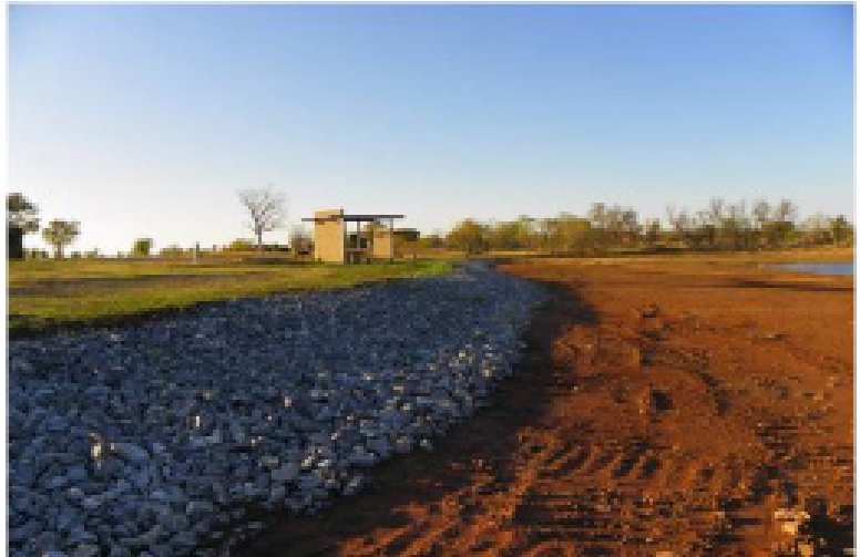
A long strip of riprap was placed in the area of the South Loop of Kiowa Park 1 at Waurika Lake in Oklahoma as part of erosion control work done while the water was low because of drought. The riprap will help prevent the loss of several campsites and the roadway, and will prevent utility lines from being exposed.
