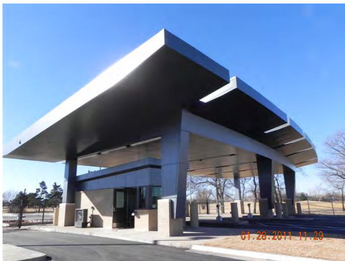
New canopy at Air Depot Gate
