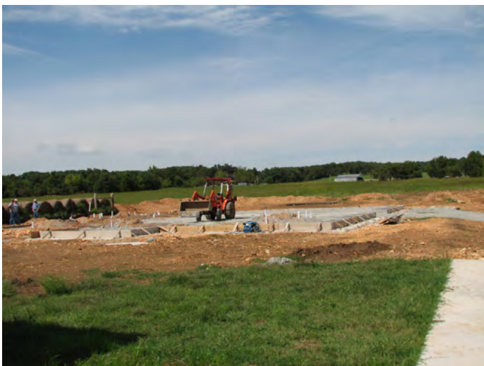
Seneca Cayuga Wellness Center foundation work
