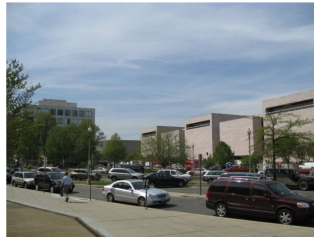
Figure 3-18: Maryland Avenue Right-of-Way and Parking
