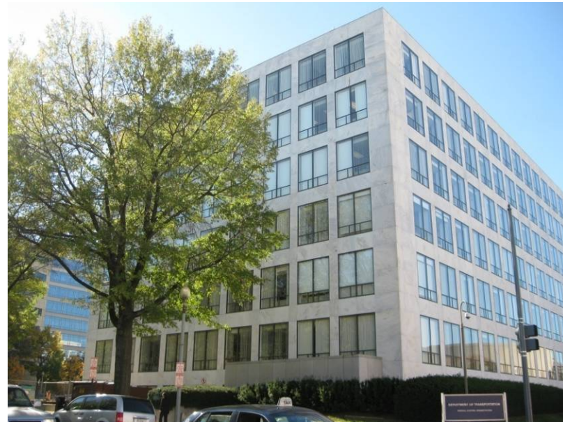
Figure 3-21: The Wilbur Wright Building and intersection of 7 th Street and Maryland Avenue located west of the Memorial site Source: AECOM, 2010
