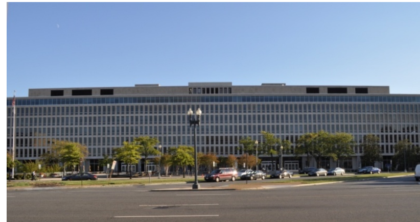
Figure 3-8 North Elevation of the Lyndon Baines Johnson Building Source: AECOM 2010
