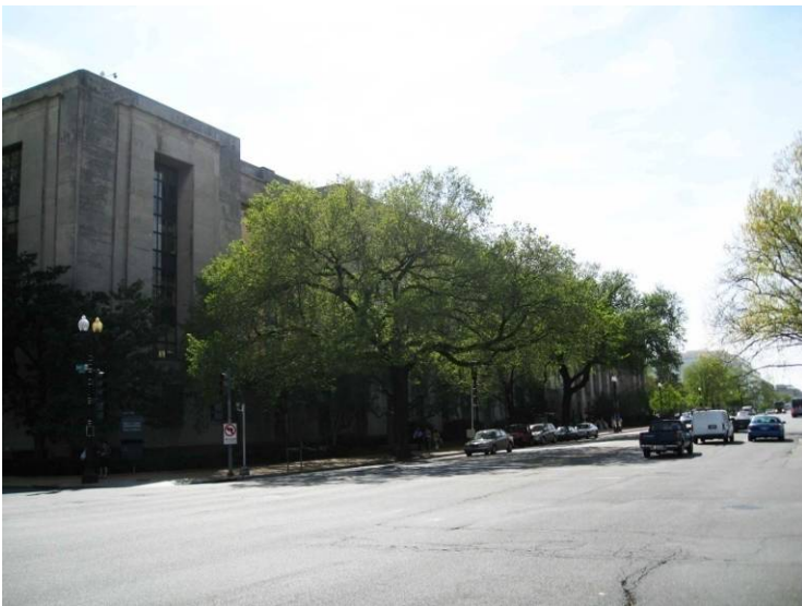
Figure 3-12: Wilbur Cohen Building Source: AECOM, 2010
