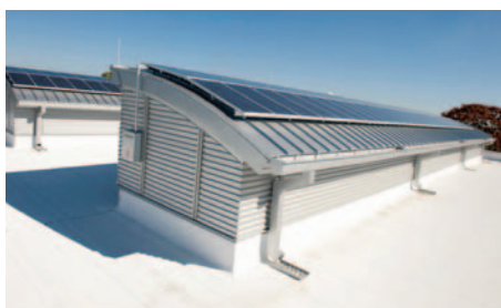
The fitness center at Tyndall Air Force Base, Florida, features a solar-generated, hot-water system and cool-roof technologies that are expected to achieve a 9% energy savings for the building. Photo from Jonathan Green, U.S. Air Force
