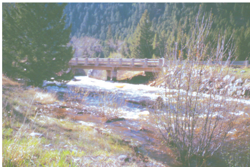
Figure 21. Boulder River below Little Galena Gulch (site 58) during spring runoff, June 1997.
