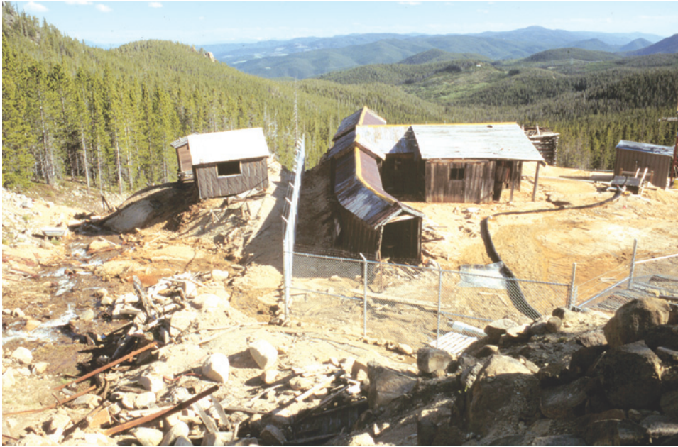
Figure 8. Crystal mine, June 1997. Acidic discharge drains from adit (out of view near lower right of photograph) to Uncle Sam Gulch on far left.
