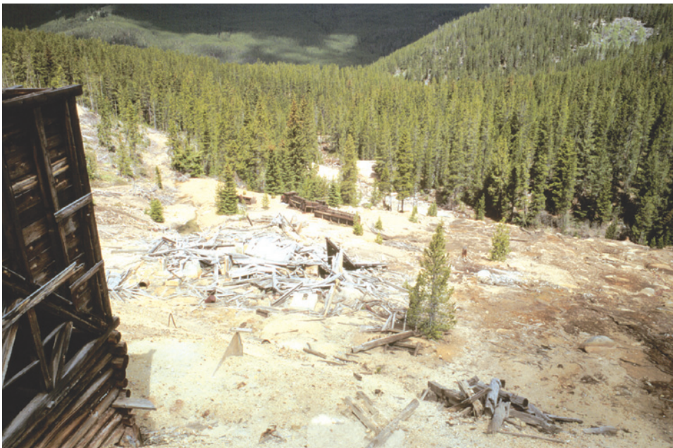
Figure 9. Bullion mine, June 1997. Primary adits are on hillslope denuded by mine wastes above Bullion Mine tributary, which flows from right to left at edge of trees at center right of photograph. Acid discharge from one adit flows downslope in lower right corner.
