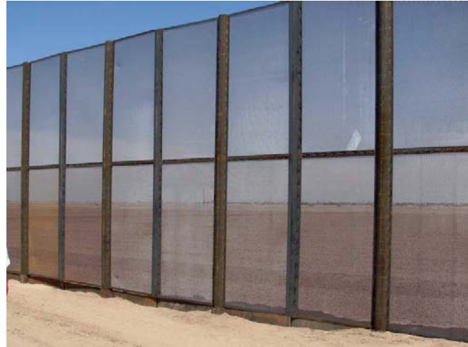
Photograph 2-1: Typical primary pedestrian fence
