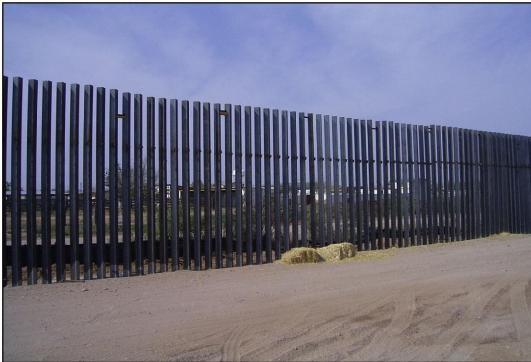
Figure B-3. Bollard Fence
