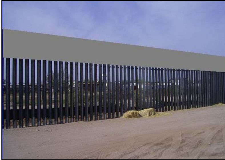
Figure 1-3. Personnel-Vehicle Fence Type 1 (PV-1)
