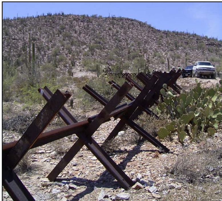
Figure 1-4. Schematic and Photograph of Vehicle Fence Type-2 (VF-2)
