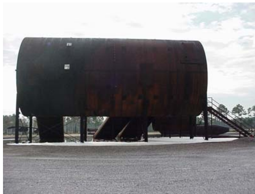
Figure 51. View of Left Side, Facing Southeast
