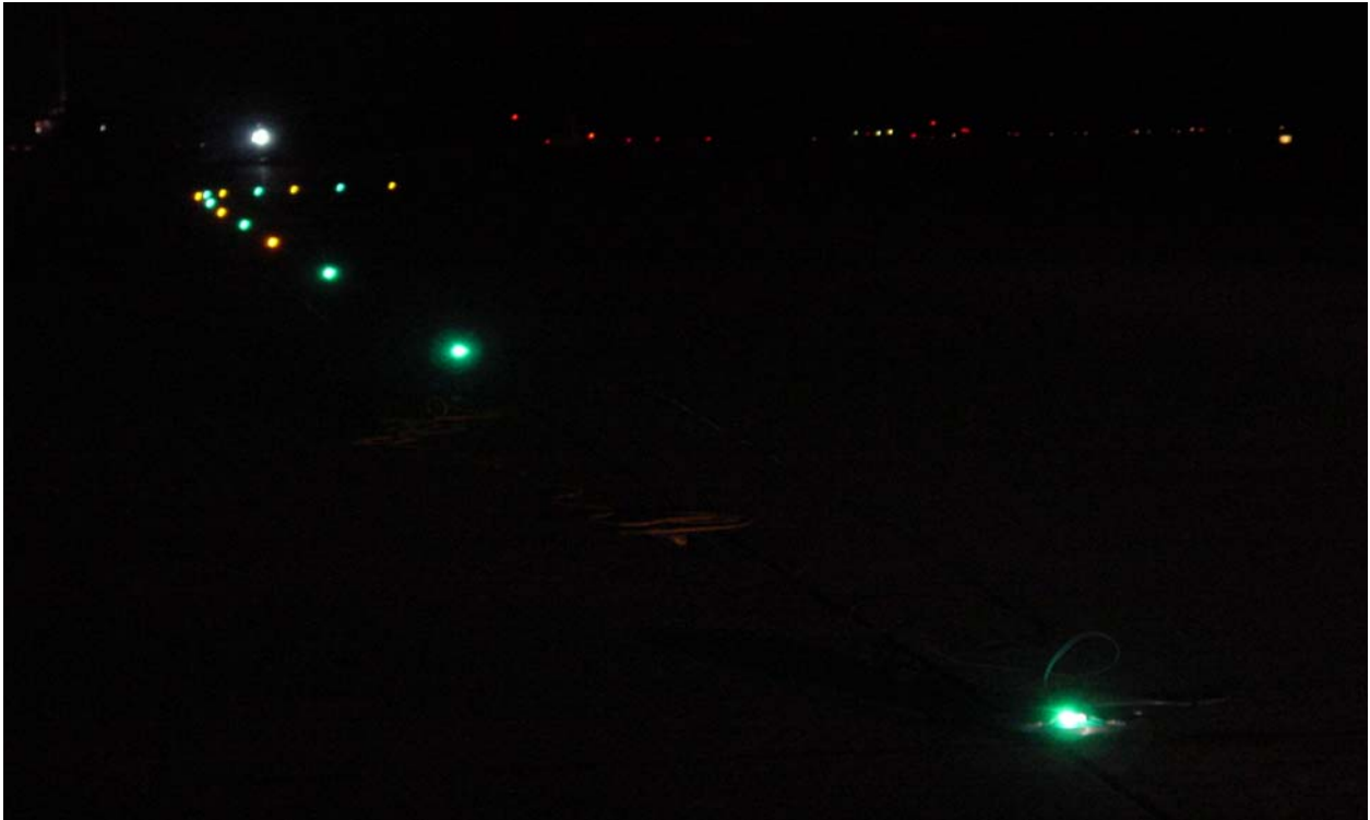
FIGURE 3. LIGHTING ARRAY AS INSTALLED FOR TEST
