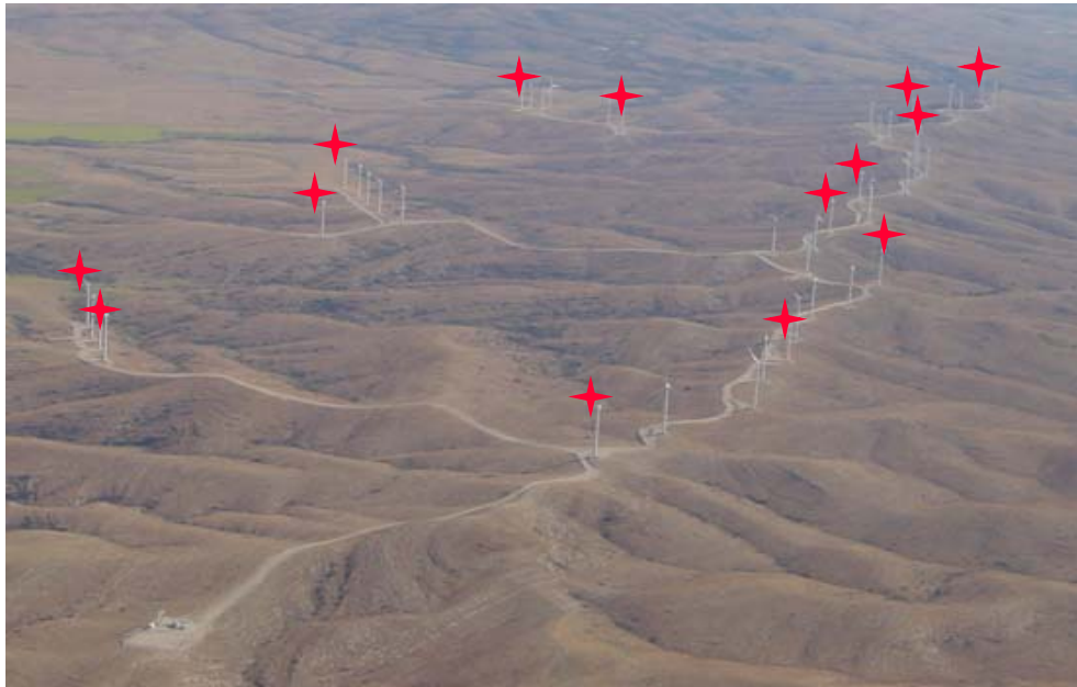
FIGURE 10. BLUE CANYON WIND FARM LIGHTING SCHEME
