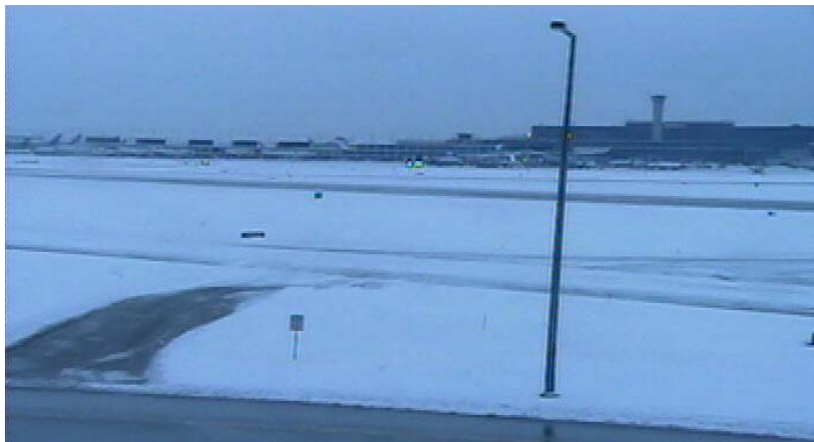
Figure 49. No Snowfall, Pavement Covered, 1/22/05, 12:00 p.m., 21°/27.1°F
