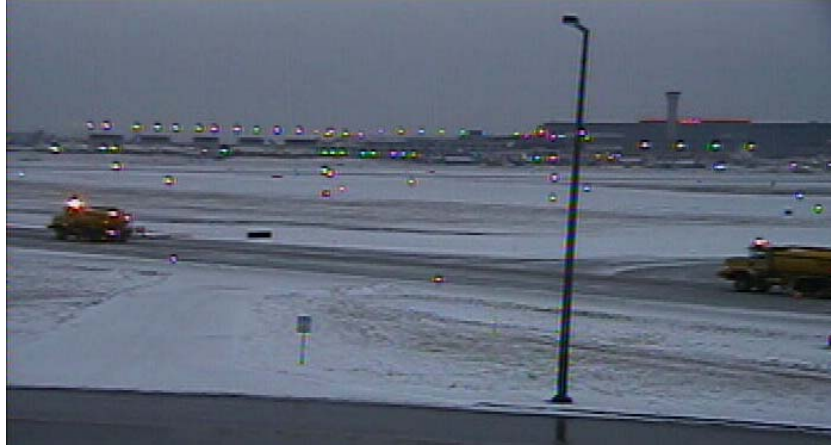
Figure 39. Deicing Agent Applied Again, 1/20/05, 4:49 p.m., 26°/27.7°F
