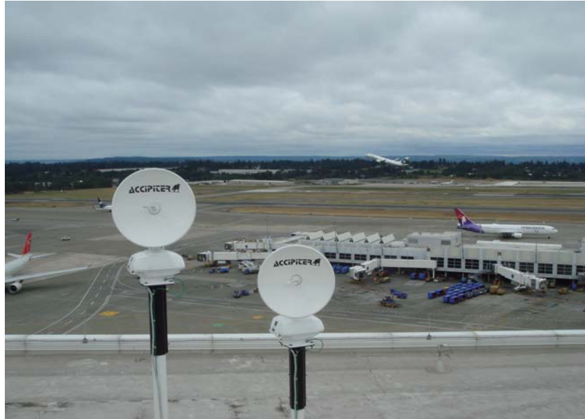
Figure 6. Parabolic Dish Antennae Mounted on the Administration Building at SEA
