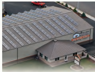
Solar roof installation funded through REAP in 2010
