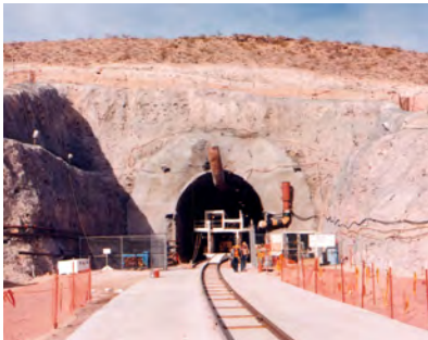
Entrance Tunnel at Yucca Mountain
