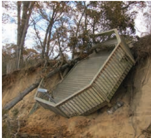
At Trustum Pond National Wildlife Refuge in Rhode Island, top, the storm breached the barrier between a freshwater pond and the Atlantic Ocean. At Target Rock Refuge on Long Island, NY, the storm dislodged an overlook deck from its foundation. (USFWS)
