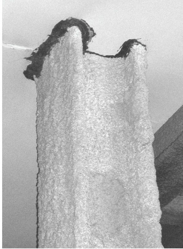
Figure 1-2 Spray-on fireproofing and smoke-seal caulking are two examples of passive fire protection.
