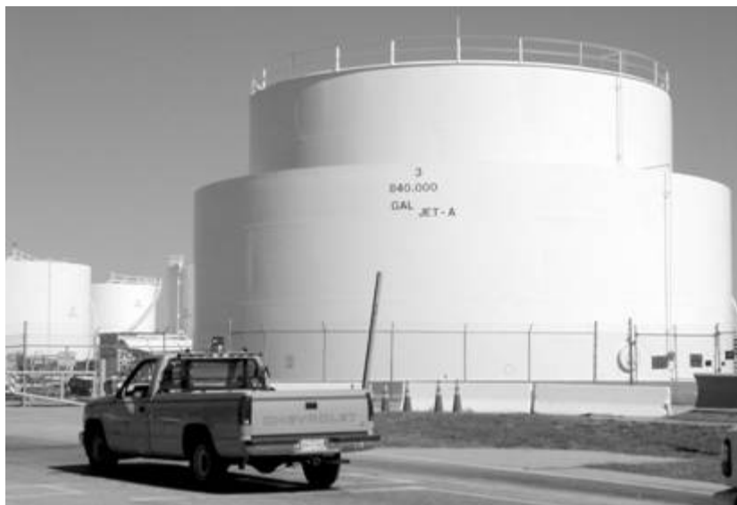
Figure 3-1(b) A Hazardous Materials Tank Farm Nearly Always is a Target Hazard
