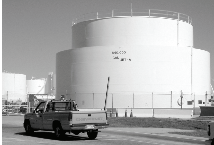
Figure 3-1(b) A Hazardous Materials Tank Farm Nearly Always is a Target Hazard
