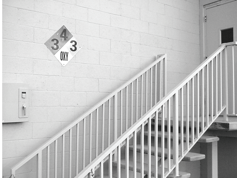
Figure 3-5 Knowing the Hazards Prior to an Event is Critical for the IC
