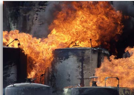
Low pressure and pressurized tanks must be adequately vented to prevent catastrophic failure when the vapors are ignited. (Kansas State Fire Marshal's Office Photo/ Steel Tank Institute and Mike Heim)
