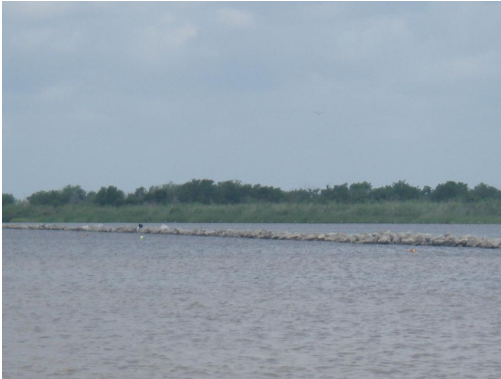
Photo 1. Typical Rock Dike
