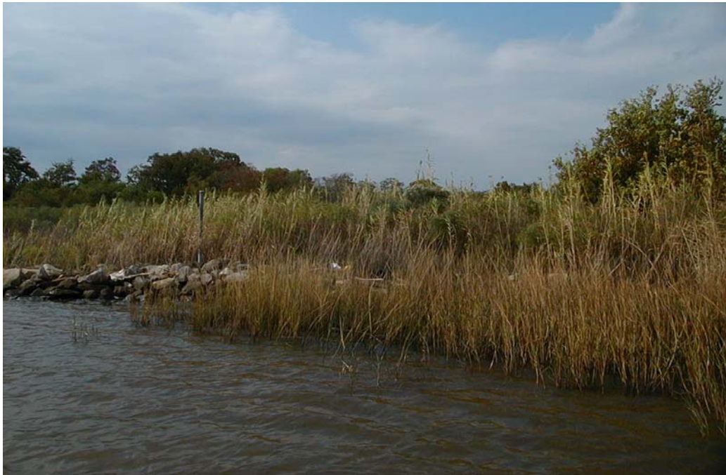
Photo 1—East tie-in at Alkali Ditch
