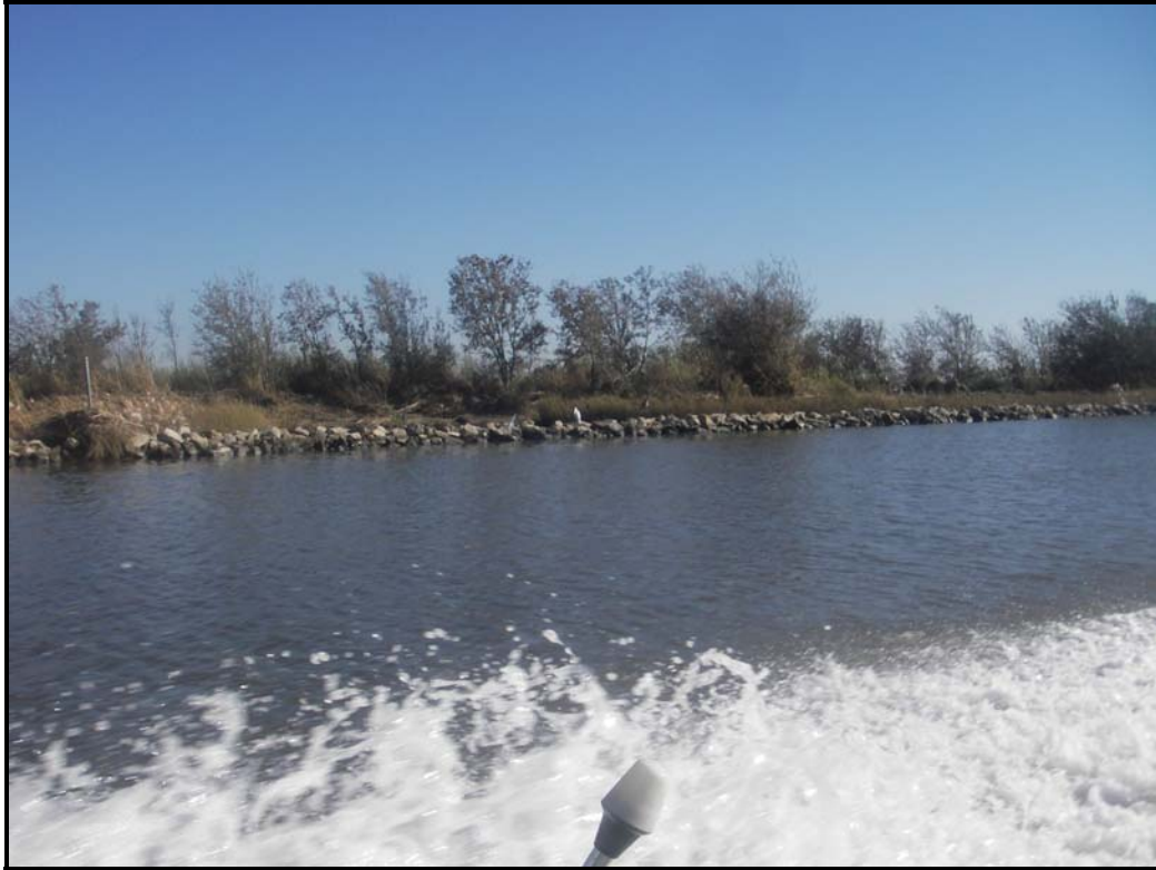
Photo No. 1, Typical rock dike
