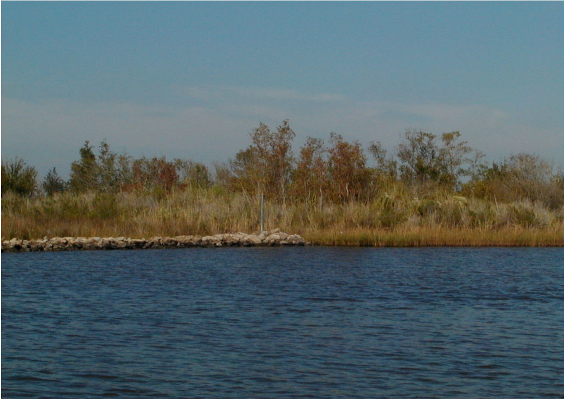
Photo 1 —East tie-in at Alkali Ditch
