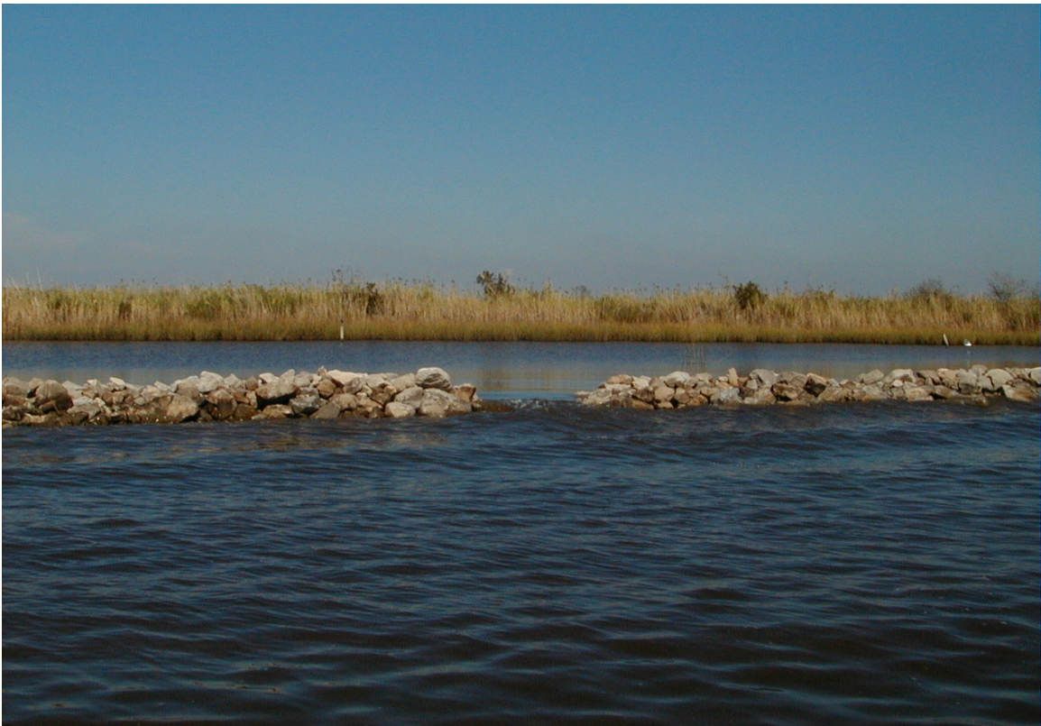
Photo 2 —vandalized area of dike
