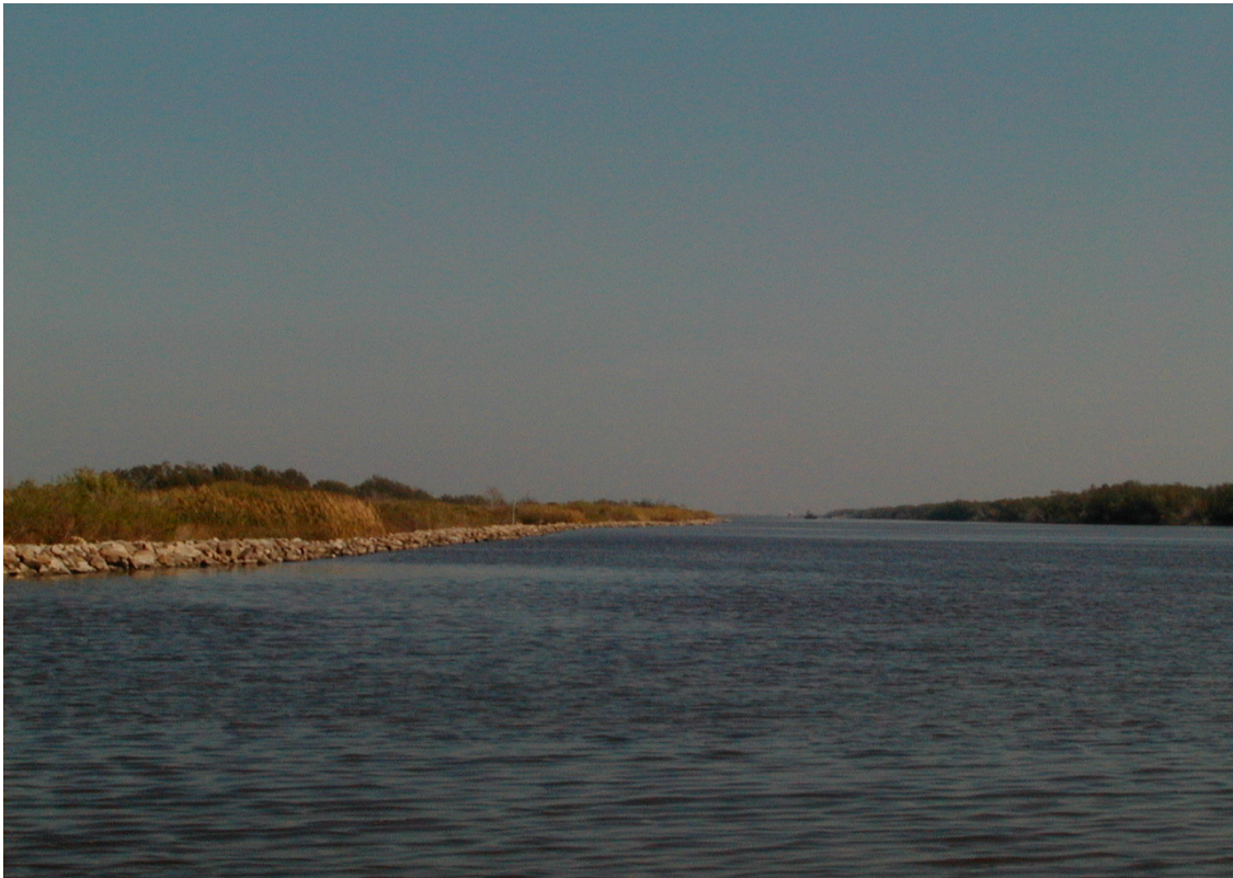
Photo 3 —typical section of dike
