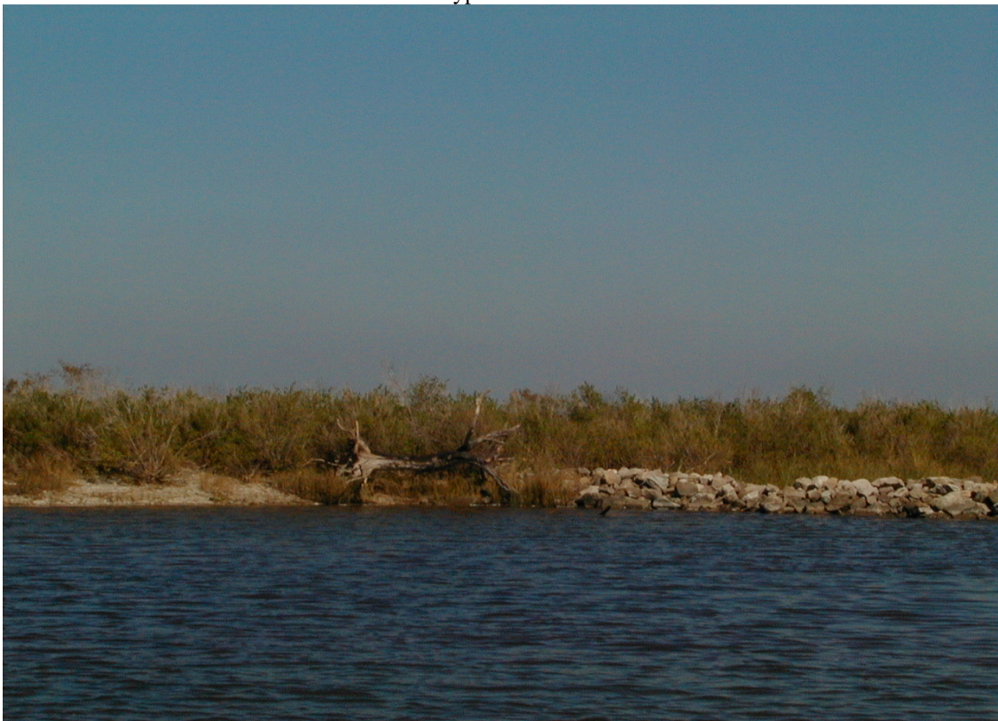
Photo 4 —western tie-in of dike
