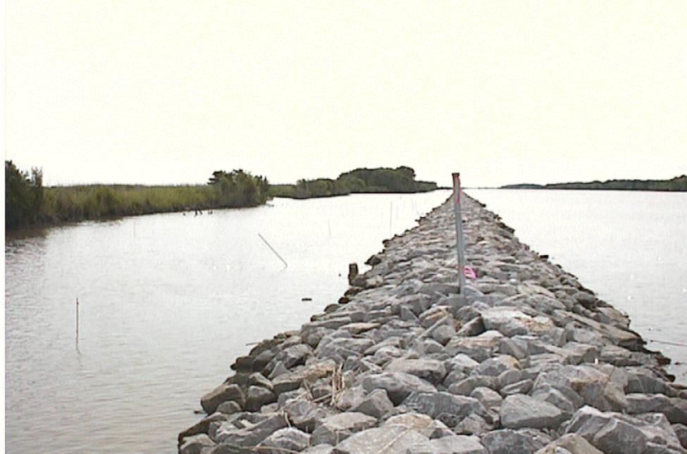
Figure 2. Photo of the rock breakwater looking W to E showing settlement plate (center), shoreline position (left side) and the GIWW Canal (right side).
