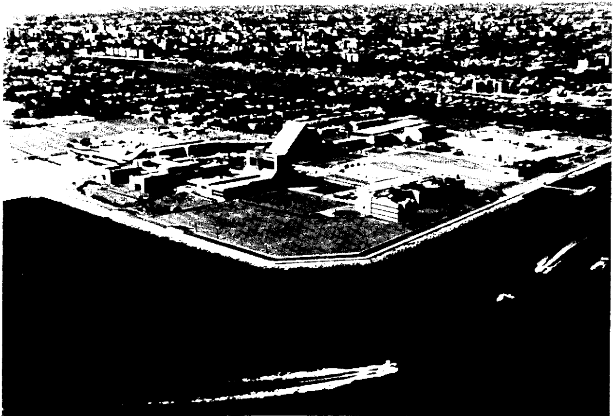
Fig. 7. Aerial site of the proposed site for marine development at Kingsborough Community College at Sheepshead Bay, Brooklyn.
