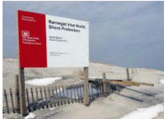
Barnegat Island Shore Protection, New Jersey (Philadelphia District)
