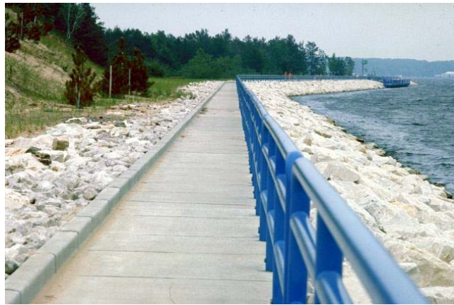
Muskegon Harbor Revetment (Detroit District)
