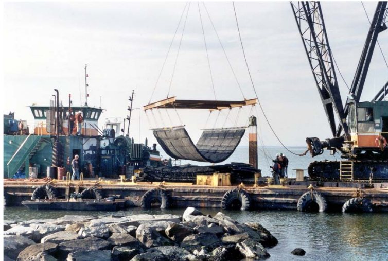
Placement of Marine Mattress (Philadelphia District)
