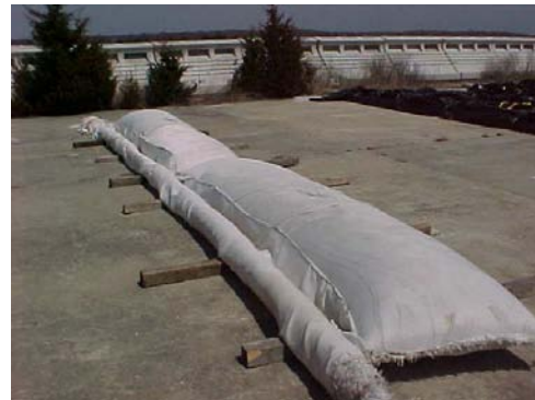
Scour Apron (Philadelphia District)
