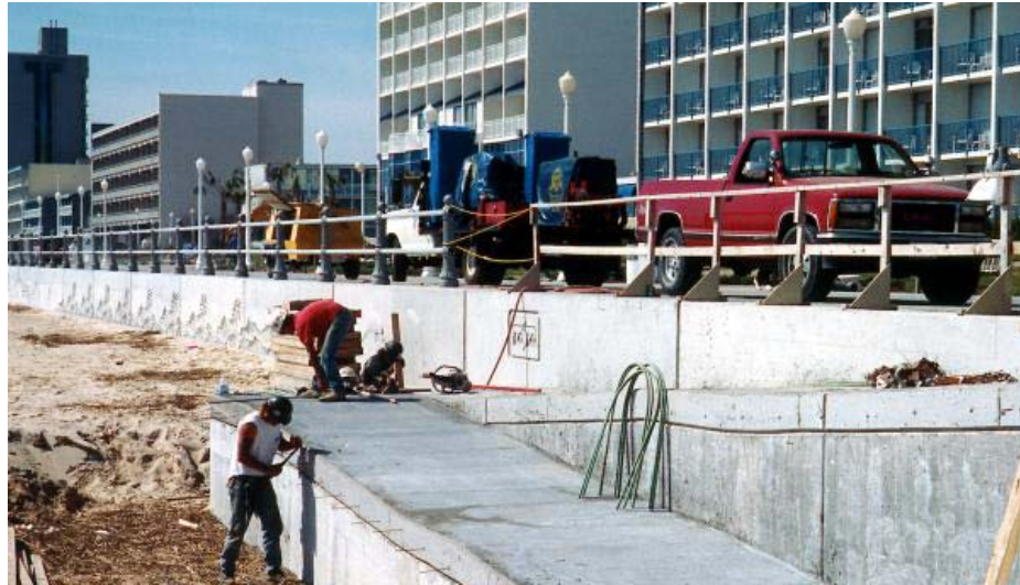
Construction the Virginia Beach Seawall, Virginia (Norfolk District)
