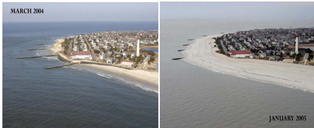
Before and After Groin Placement at Cape May Point, New Jersey
