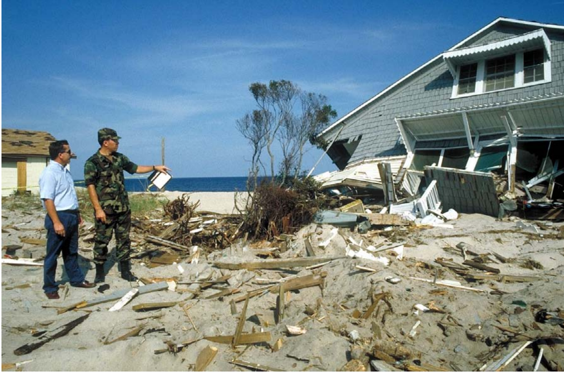
Topsail Beach, North Carolina after Hurricane Fran (Anthony Bley, Philadelphia District)
