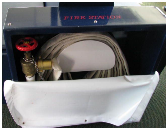
Firemain System on a Passenger Vessel.
