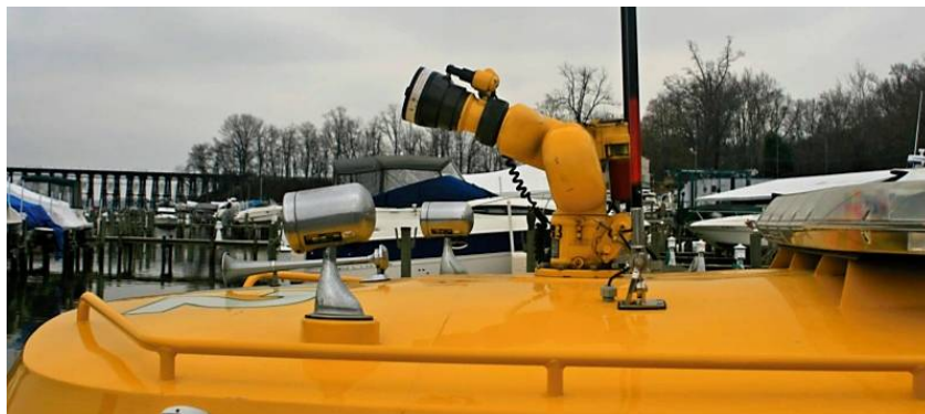
Firemain System on a Fire Boat.
