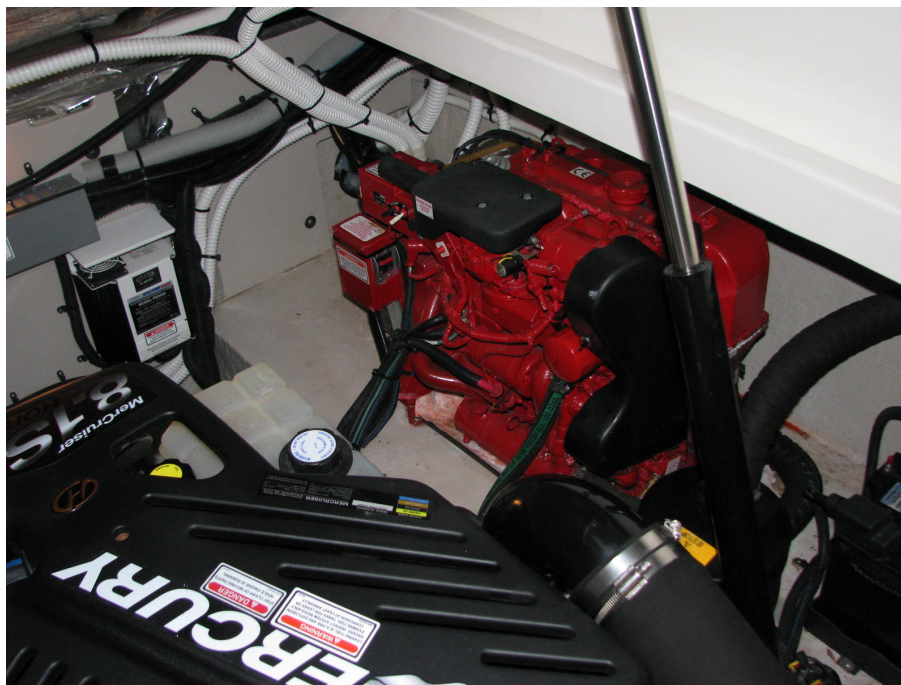
The Generator on a Fire Boat
