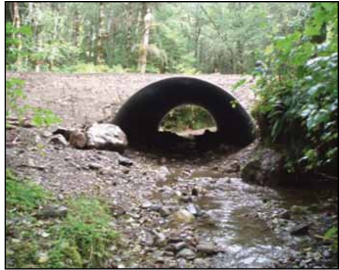
Figure 4.11—Fish passage culvert at Olympic National Forest. (Photo courtesy of USDA Forest Service, Olympic National Forest.)
