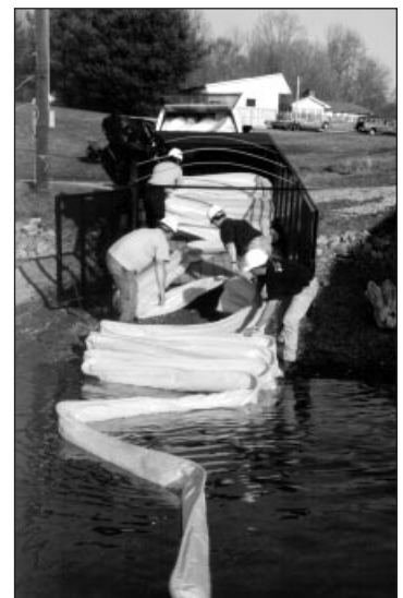
TVA crews work to contain Colonial Pipeline's diesel-fuel spill along the Knoxville waterfront.
