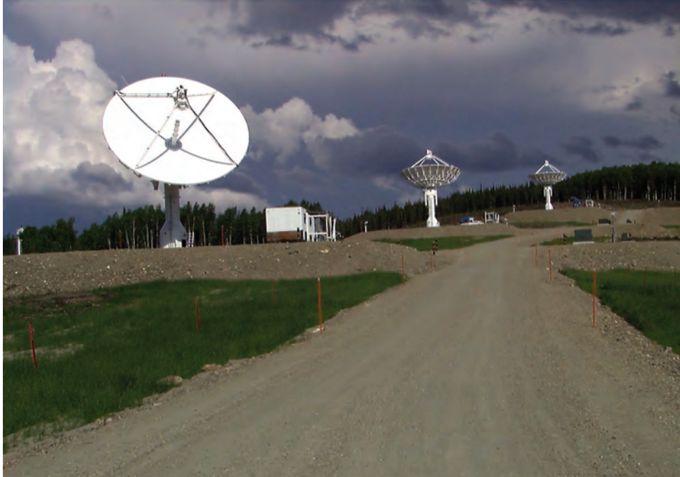
Satellite antennae at Fairbanks Alaska Satellite Operations Facility (FSOF)
