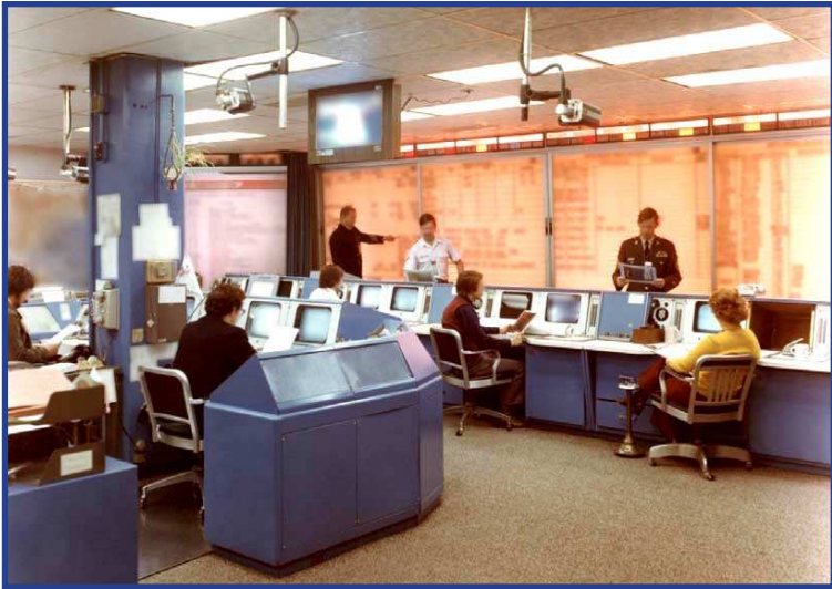
Operations Watch Area after modernization with improved computer screen displays
