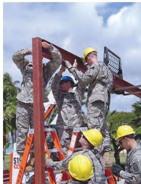
U.S. Army Reserve engineer Soldiers lay out (left) and assemble (above) the iron framework for the Battery Randolph parapets during the Soldiers' 21-day annual training requirement. More than 310 reservists from the 980th Engineer Battalion, 420th Engineer Brigade and the 416th Theater Engineer Command participated in the 63-day "Operation Akamai Builder." Courtesy photos
