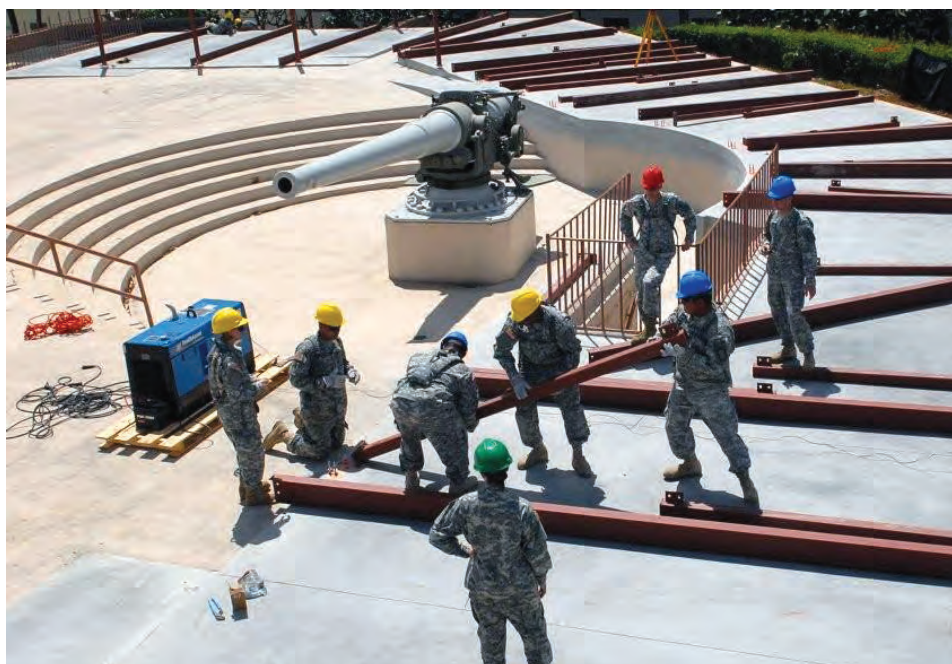
U.S. Army Reserve engineer Soldiers lay out (left) and assemble (above) the iron framework for the Battery Randolph parapets during the Soldiers' 21-day annual training requirement. More than 310 reservists from the 980th Engineer Battalion, 420th Engineer Brigade and the 416th Theater Engineer Command participated in the 63-day "Operation Akamai Builder." Courtesy photos
