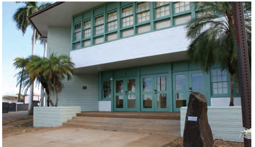
A view of the Aloha Center’s new entrance facade that now resembles the building’s original design from the 1940s. Photo by Dino W. Buchanan
